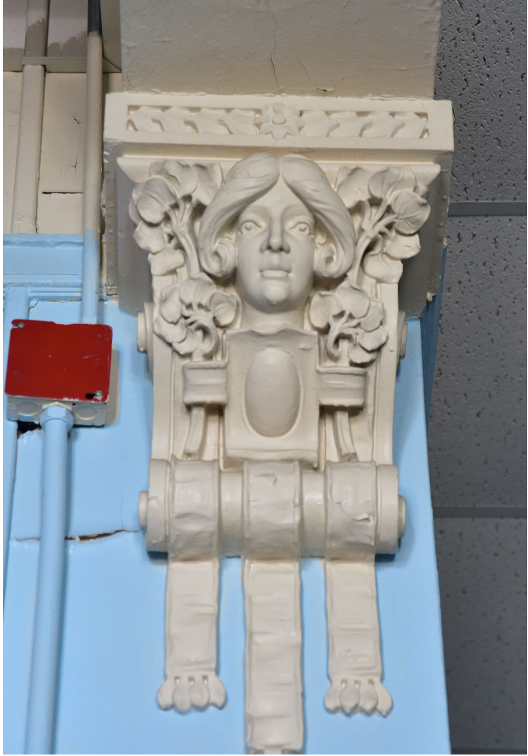
Figure 17. Detail photo of corbels in 1912 section. Source: f-stop Photography, December 2020.
