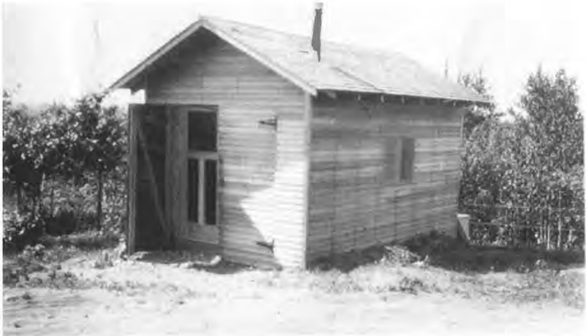
Figure 2. A June 1929 photograph of the 12' x 16' warehouse (i.e., storage building) about one year after construction. Its poured concrete foundation (Photo 16) is located about 50' west of the tower. From 1941-1956 the building served as the office for the Pequot ranger district. In the foreground is the south side of the access road loop (photo by the Minnesota Forest Service, Minnesota Dept. of Conservation, Forestry Division Records, Minnesota Historical Society).
