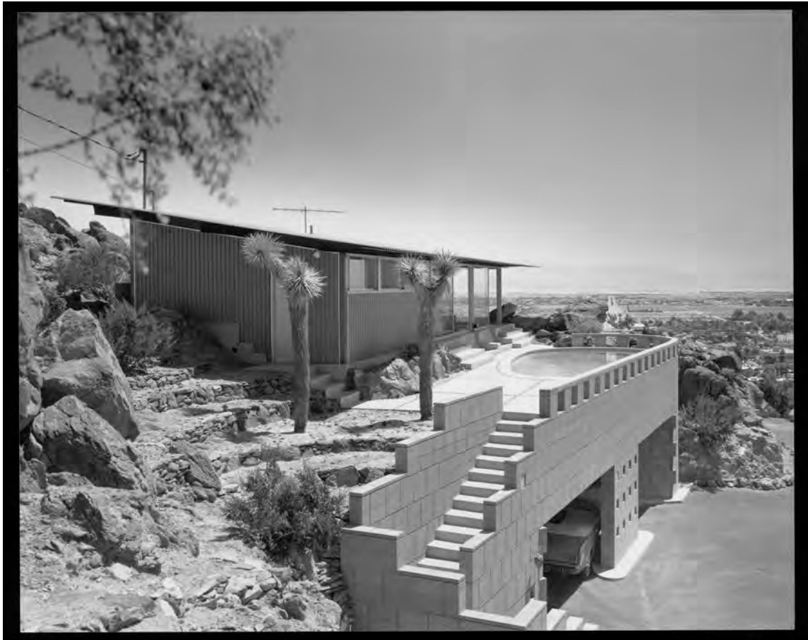
Figure 2. West and south elevations, looking northeast, 1965.
