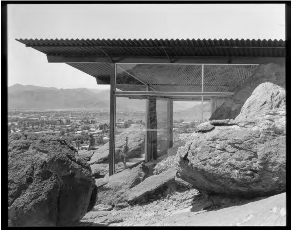
Figure 4. North elevation, looking south, 1965.
