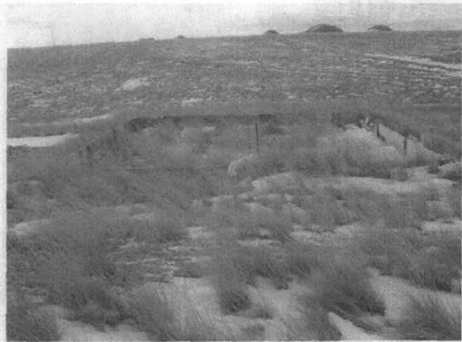
Sludge Drying Bed (T-804), contributing, view to south.
