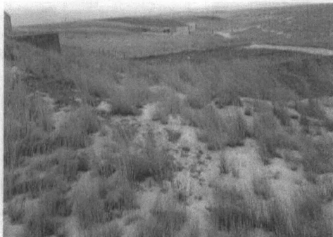
Sprinkling Filter (T-802), contributing structure, view to southeast.
