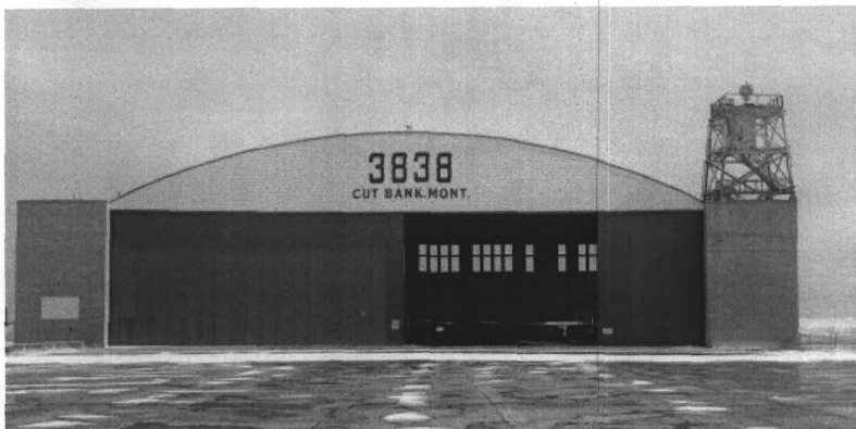
Hangar T-501, c. 1950. View to east.
