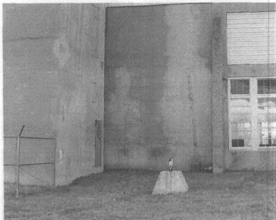
Control Tower Footings (T-502), contributing site, view to north.
