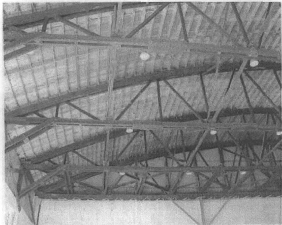
Hangar (T-501) rafters.
