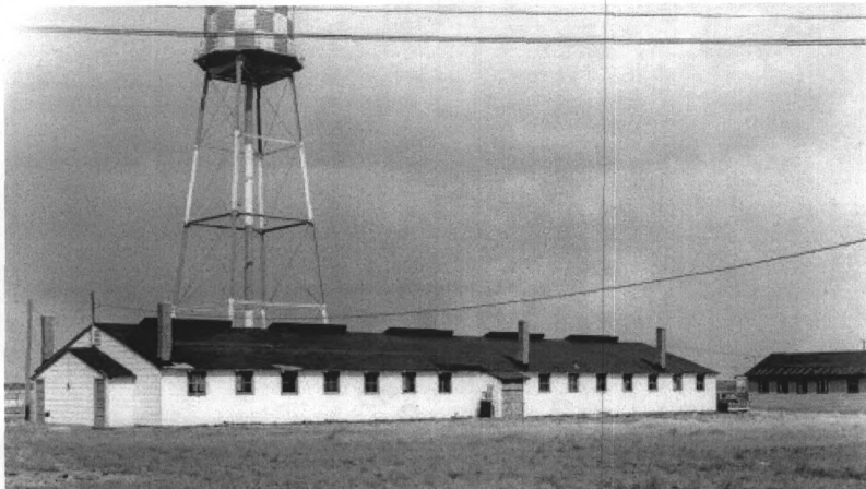
Recreation Hall T-131, c. 1950. View to northeast.
