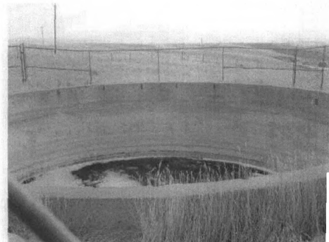
Imhoff Cone (T-801), contributing structure, view to southeast.
