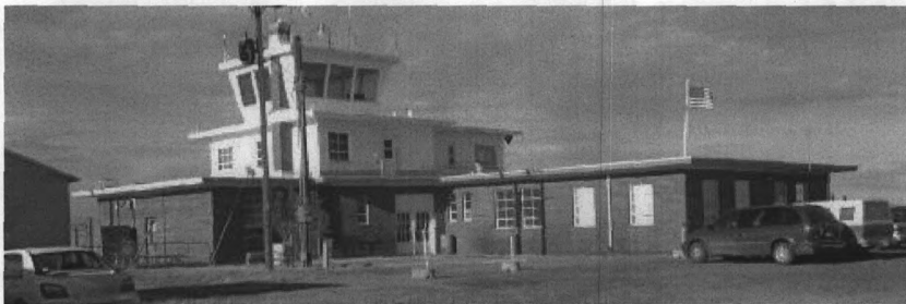
Cut Bank Municipal Airport 1948 Terminal Building, contributing building, view to the northwest.
