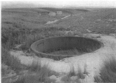
Secondary Clarifier (T-803), contributing, view to southeast.
