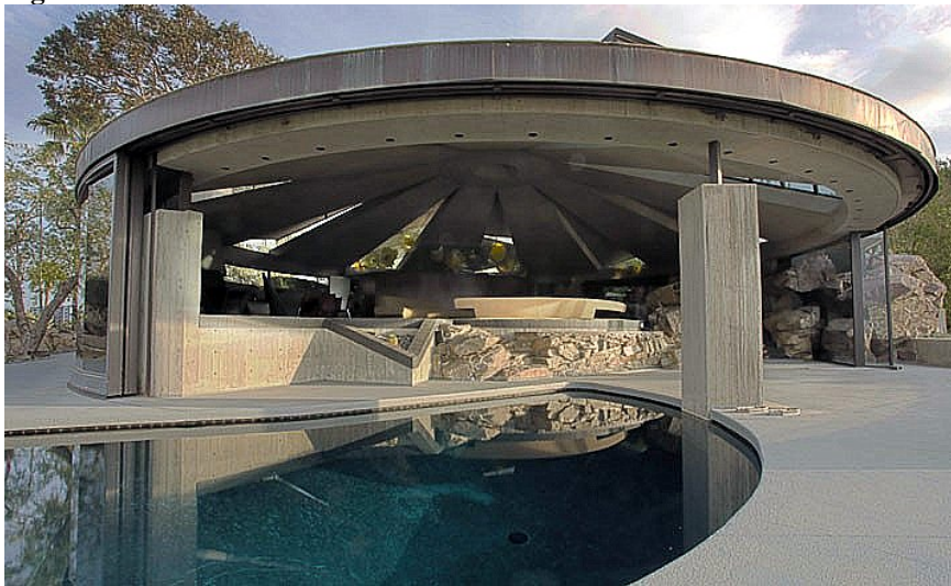
Detail of roof structure, facing south (Photo credit: Coronare Modestus Faust, photographed in 2011)
