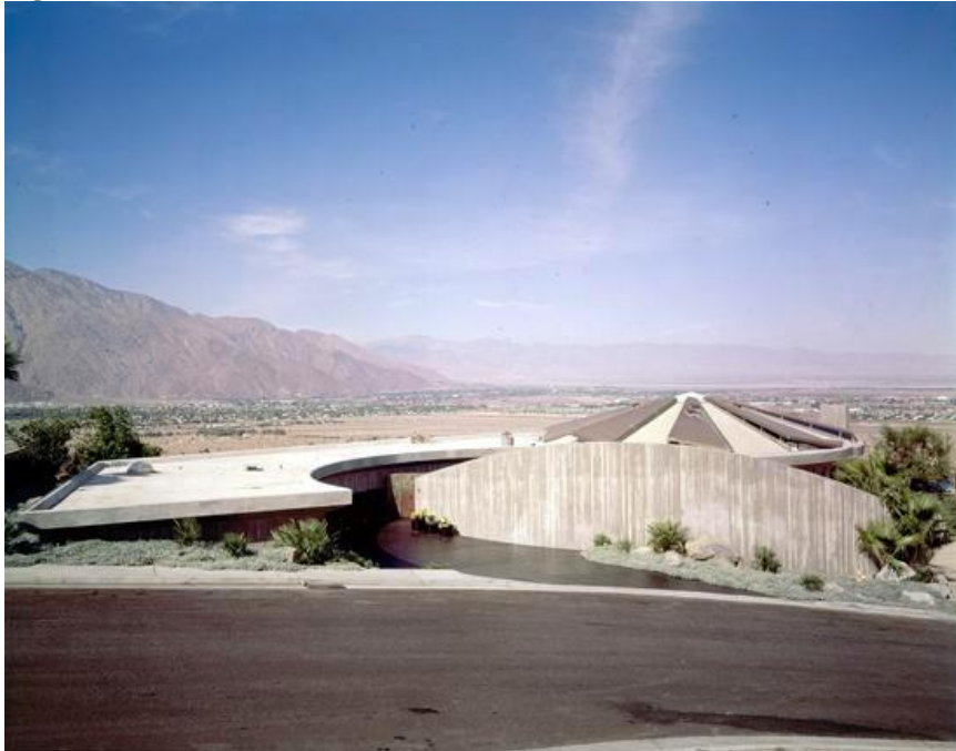
View of primary façade, facing northwest (Photo credit: Coronare Modestus Faust, photographed in 2011)
