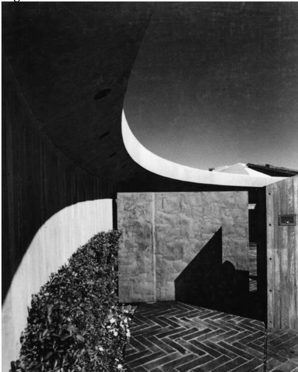
Detail of entry gate, facing northwest (© The John Lautner Foundation, courtesy of Frank Escher, date of photograph unknown)
