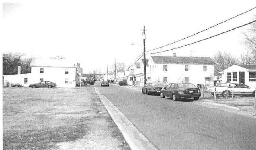
24. Pine Street Neighborhood Historic District, Park Lane looking northwest, Cambridge, Dorchester County, Maryland
