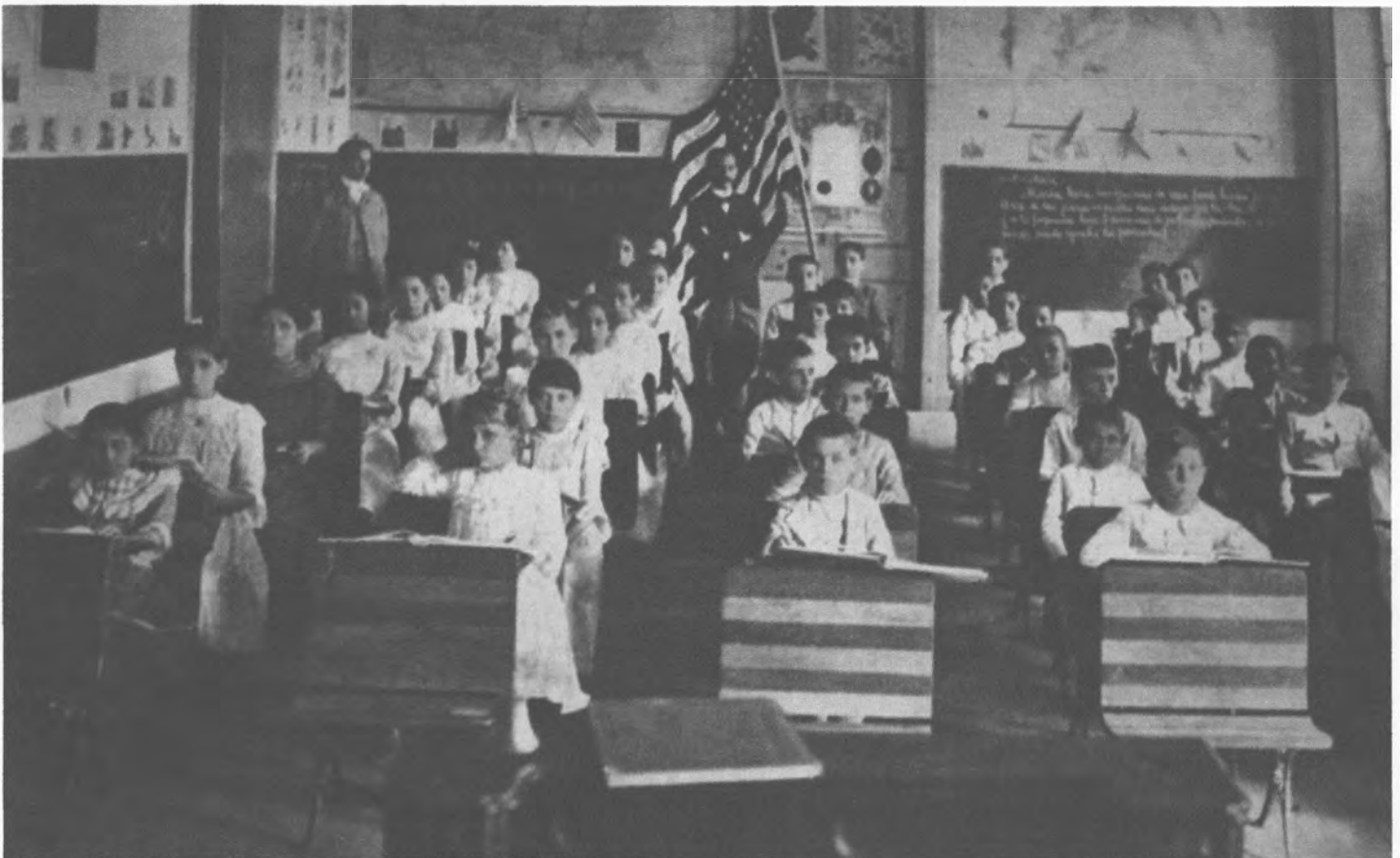
Fig. 2: Classroom in Mayaguez graded school. Source: AGPR, Annual Report of the Governor of Puerto Rico, 1902-1903.
