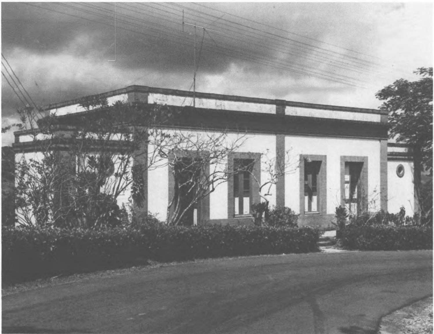
Fig. 7: "Casilla de Peón Caminero", Guayama. These prototypes were considered initially for school buildings. Source: Casillas de Caminero, by Carlos M. Colón Torres, 1961.
