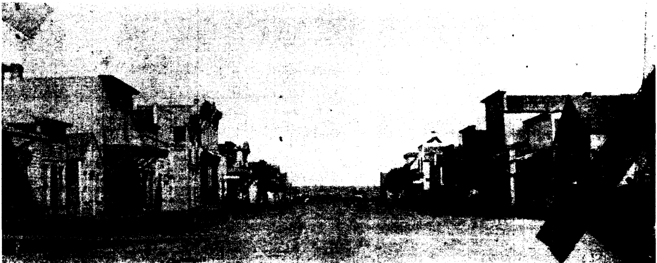
First generation buildings along Ashton's Main Street in northwest Iowa, 1885. Ashton is a railroad town in which the Main Street was drawn perpendicular to the tracks. Note the mix of one and two story buildings; the prominence of false-front pediments, and the drop-down wooden panels that provided both climate control and overnight security. From Growing Together, 24.
