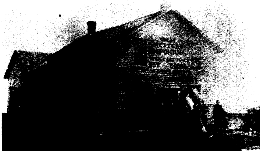
Ossian's "Great Western Emporium," in northeast Iowa in 1860. The gable-end front is clad in milled drop siding, while the less formal sides are covered with cheaper board-and-batten siding. The signage painted across the façade advertises "STAPLE AND FANCY... DRY GOODS... CLOTHING, PAT. MEDICINES, BOOTS & SHOES... HARDWARE, CROCKERY ETC." The store appears to be connected at the rear to another building, perhaps the storekeeper's residence. From SHSI, IC; reprinted in Bennett, 78.
