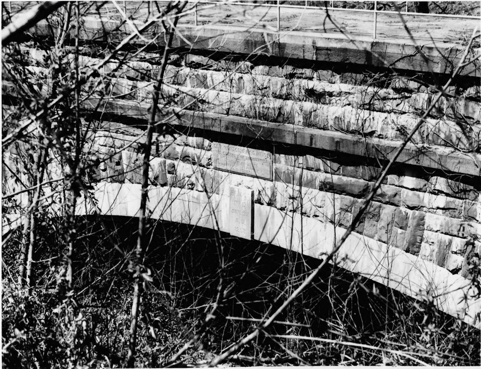
Washington Aqueduct, Bridge No. 3, Washington, D.C.
