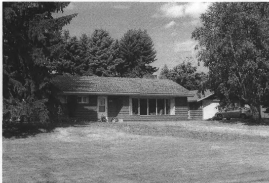
2. East façade of house and garage looking northwest.
