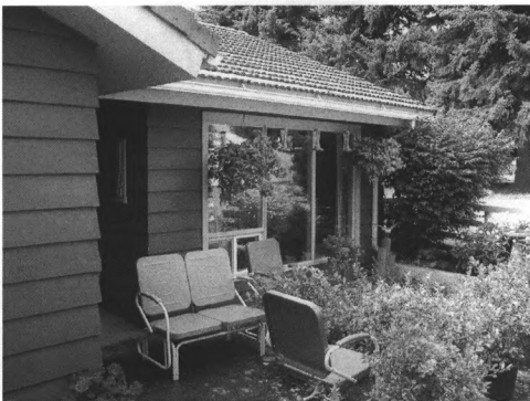
7. North elevation of west wing looking southwest.
