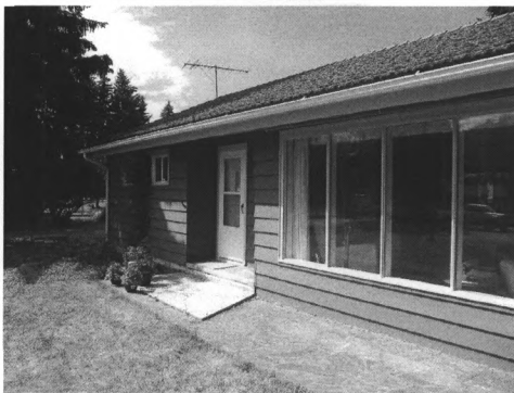
3. Detail of east façade of house looking southwest.
