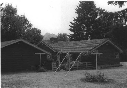
6. West elevation of garage, and west and north elevations of house looking southeast
