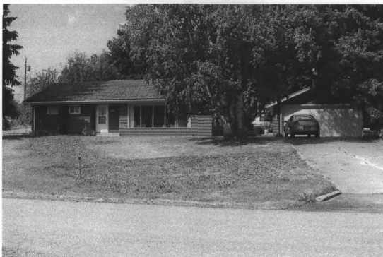
1. East façade house and garage looking west.
