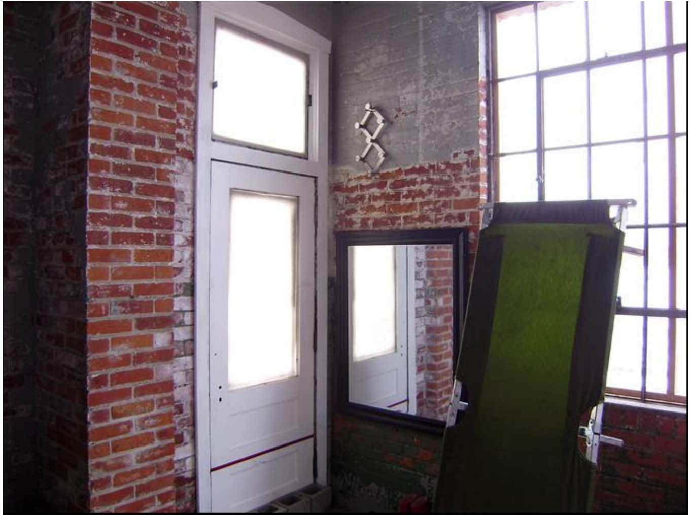
Photo 0020. Interior of operator's office door. View to southeast.
