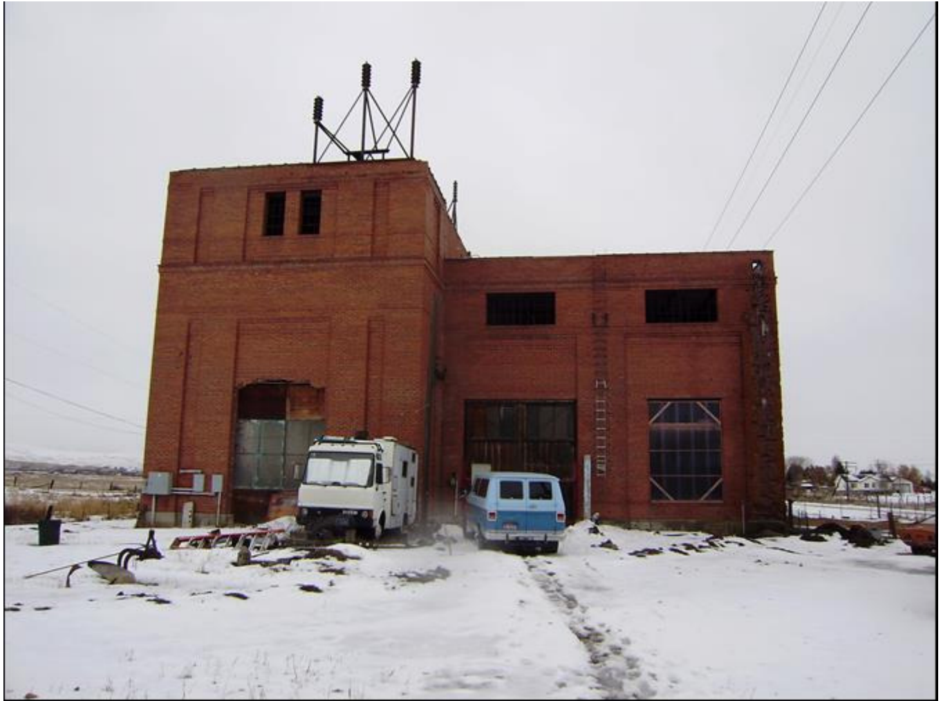
Photo 0005. West elevation. View to the south-southeast.
