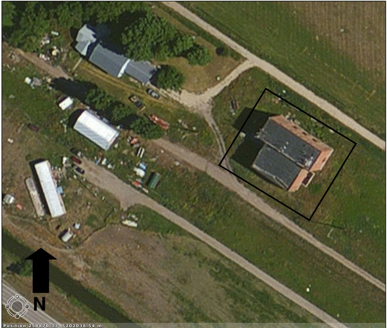
Aerial view showing Milwaukee Road Railroad Substation No. 10 (Primrose Substation). Substation located on right side of photograph encircled by black box.
