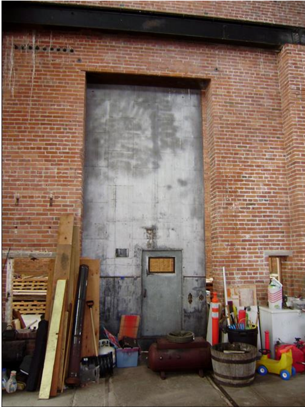
Photo 0019. Detail of interior steel partition door. View to north.
