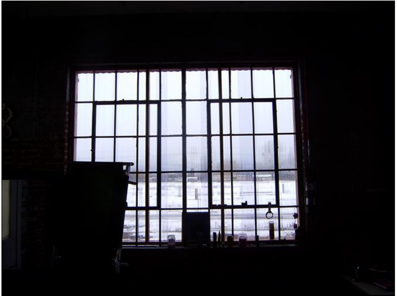
Photo 0021. Detail of operator's office window with muntins. View to southwest.
