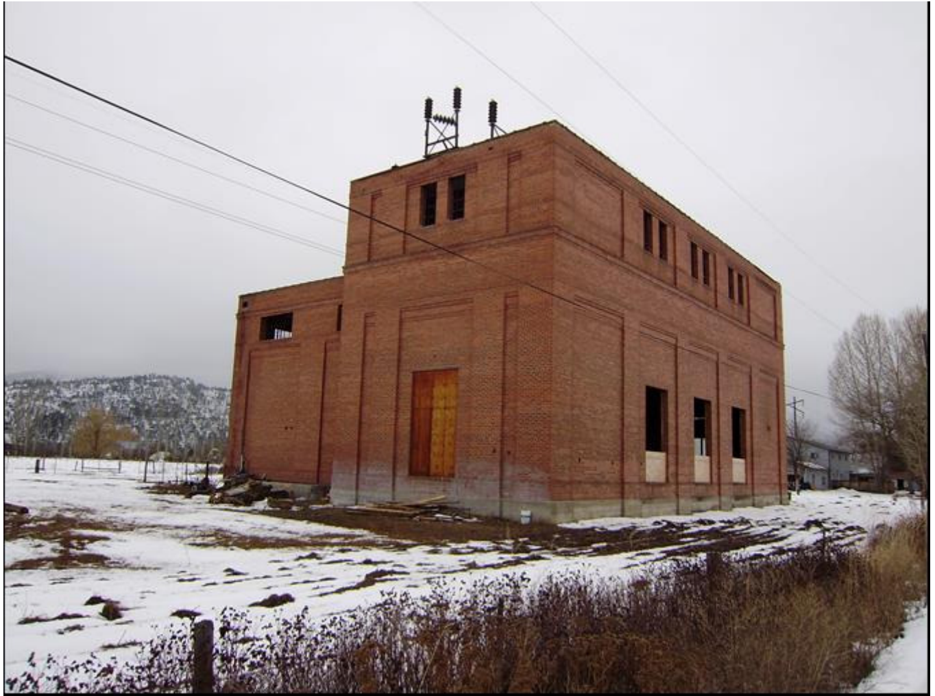
Photo 0003. East and north elevations. View to the southwest.
