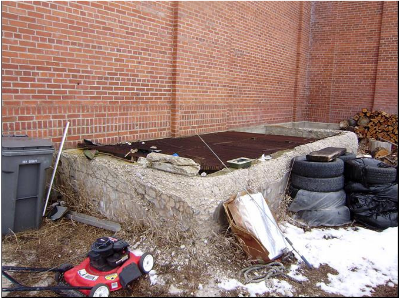
Photo 0016. Detail of ventilation pit. View to north.
