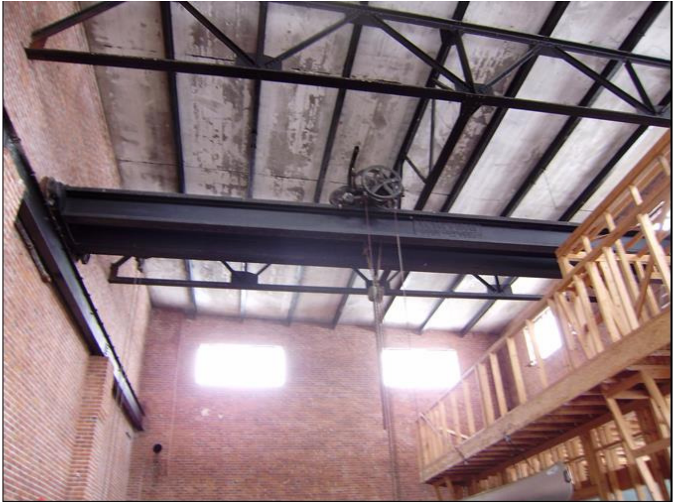
Photo 0018. Detail of interior crane. View to the east.
