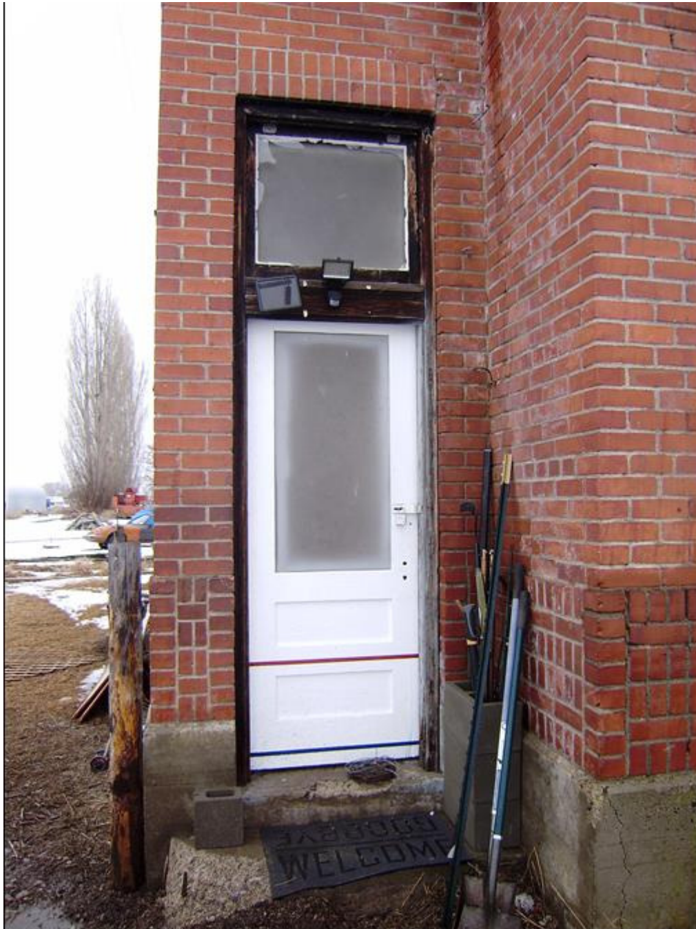
Photo 0010. Detail of entry to operator's office. View to west-northwest.
