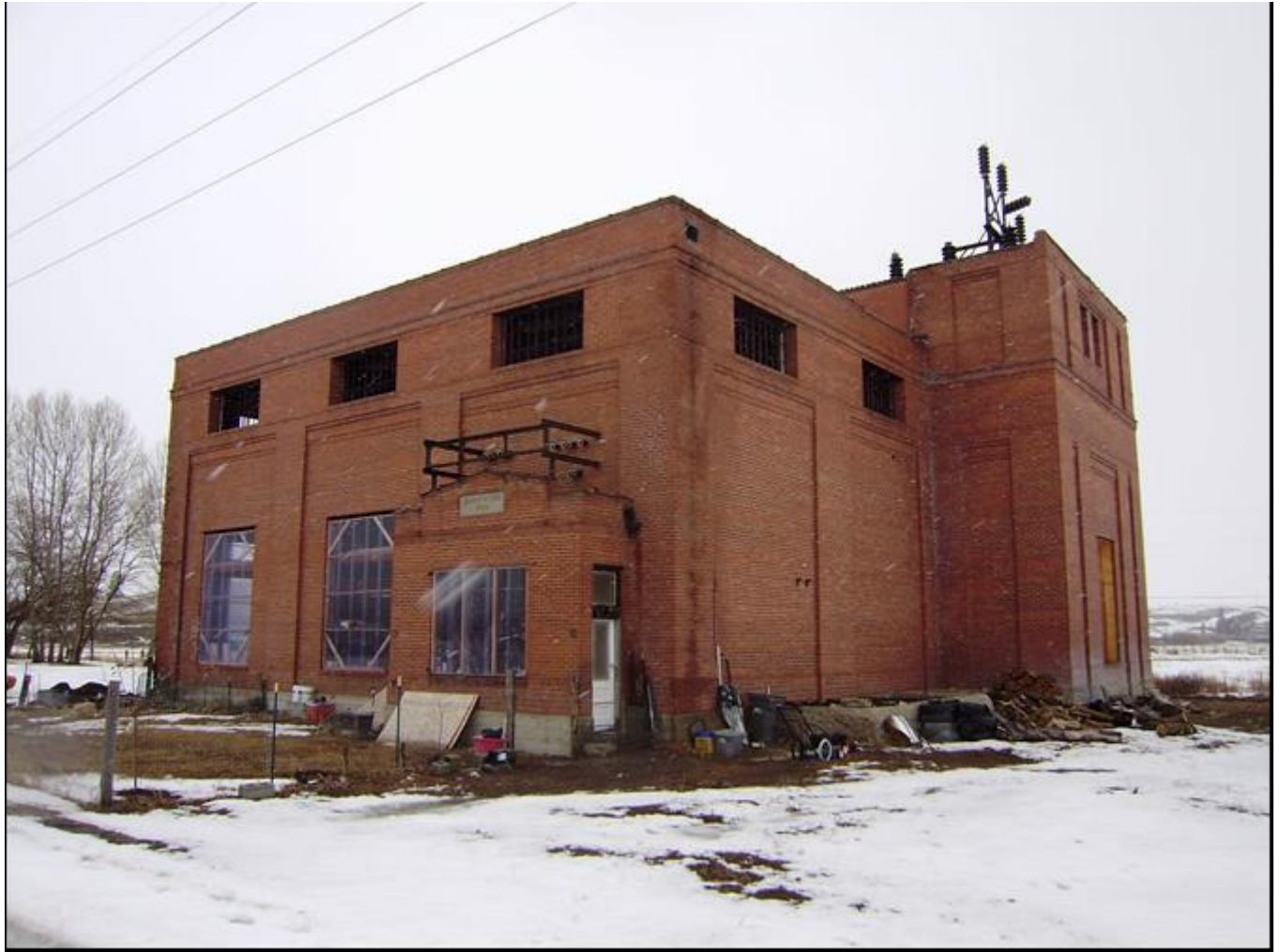
Photo 0002. Façade overview. View to north-northwest.
