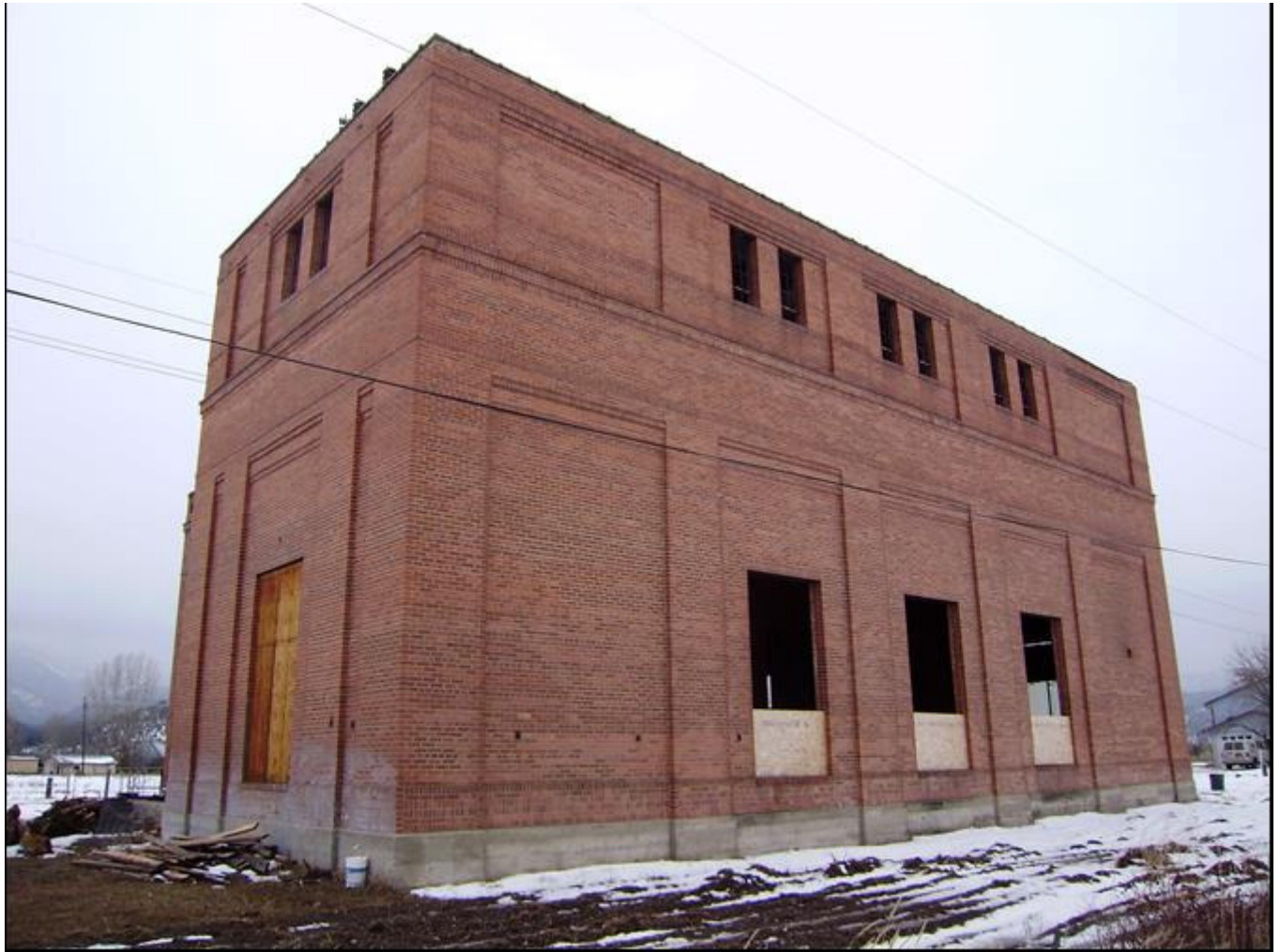
Photo 0011. North and east elevations. View to southwest.
