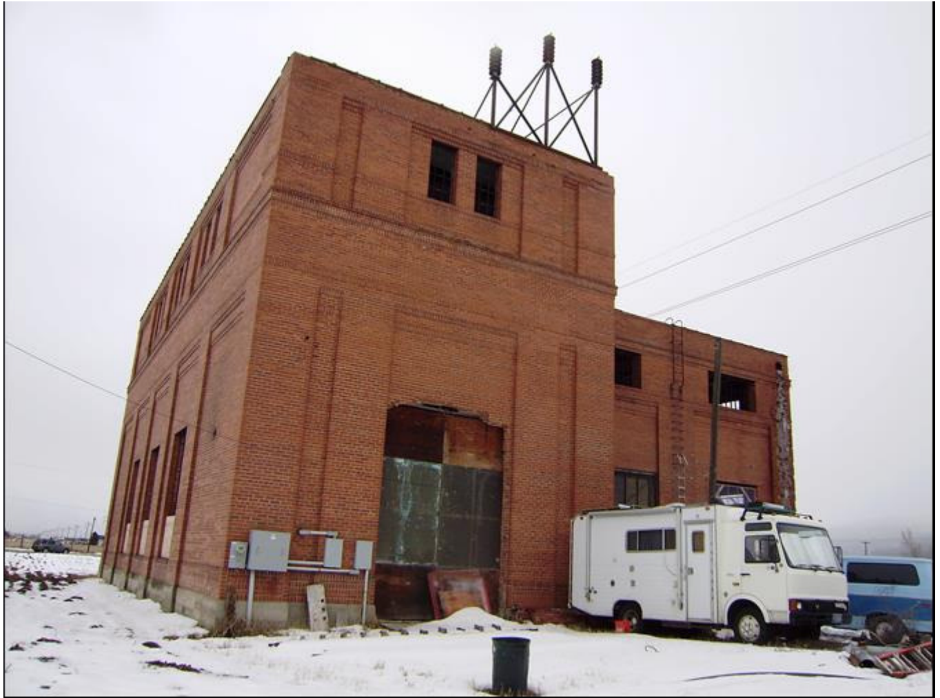
Photo 0012. North and west elevations. View to east-southeast.
