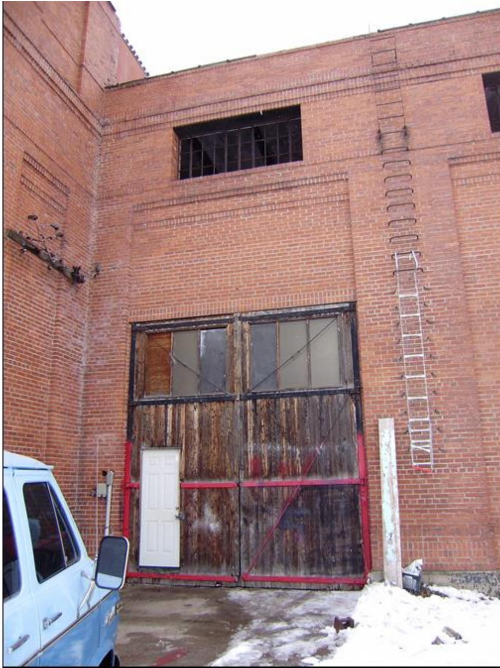
Photo 0014. Detail of bay entry on west elevation. View to southeast.
