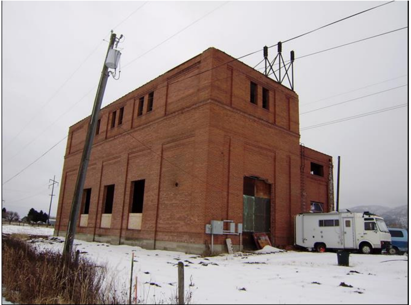
Photo 0004. North and west elevations. View to the southeast.
