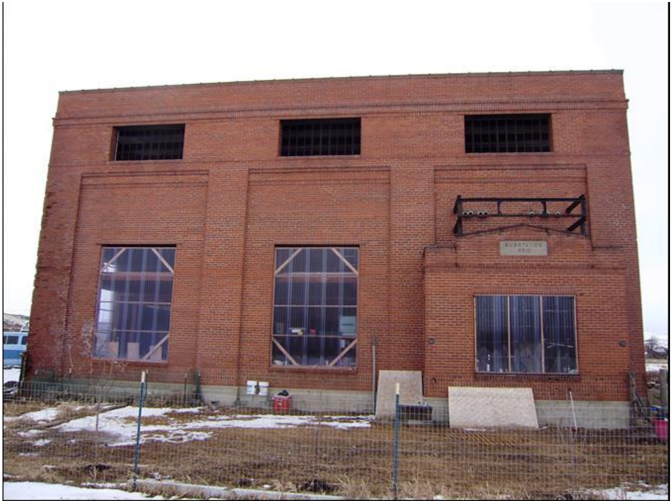
Photo 0007. Façade (south elevation). View to the northeast.
