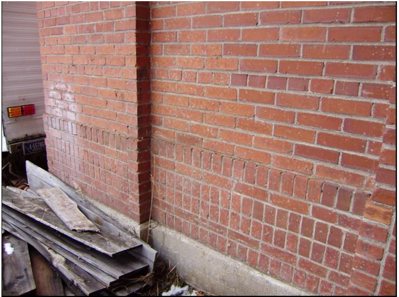
Photo 0015. Detail of brick water table. View to northeast.
