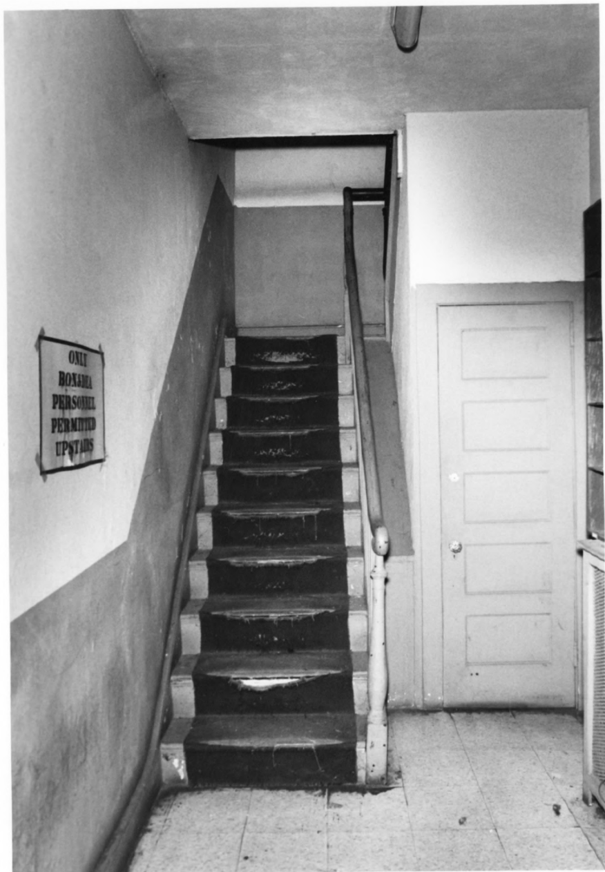
ESSEX COUNTY JAIL NJ ESSEX COUNTY PHOTO 8 OF 9
