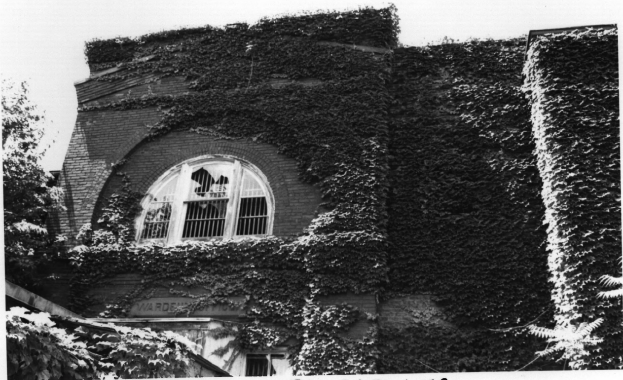
ESSEX COUNTY JAIL NJ ESSEX COUNTY PHOTO 6 OF 9
