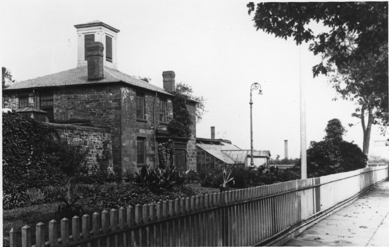
ESSEX COUNTY JAIL NJ ESSEX COUNTY PHOTO 3 OF 9
