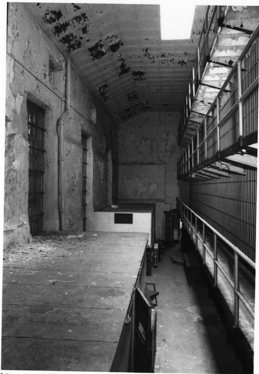
ESSEX COUNTY JAIL NJ ESSEX COUNTY PHOTO 9 OF 9
