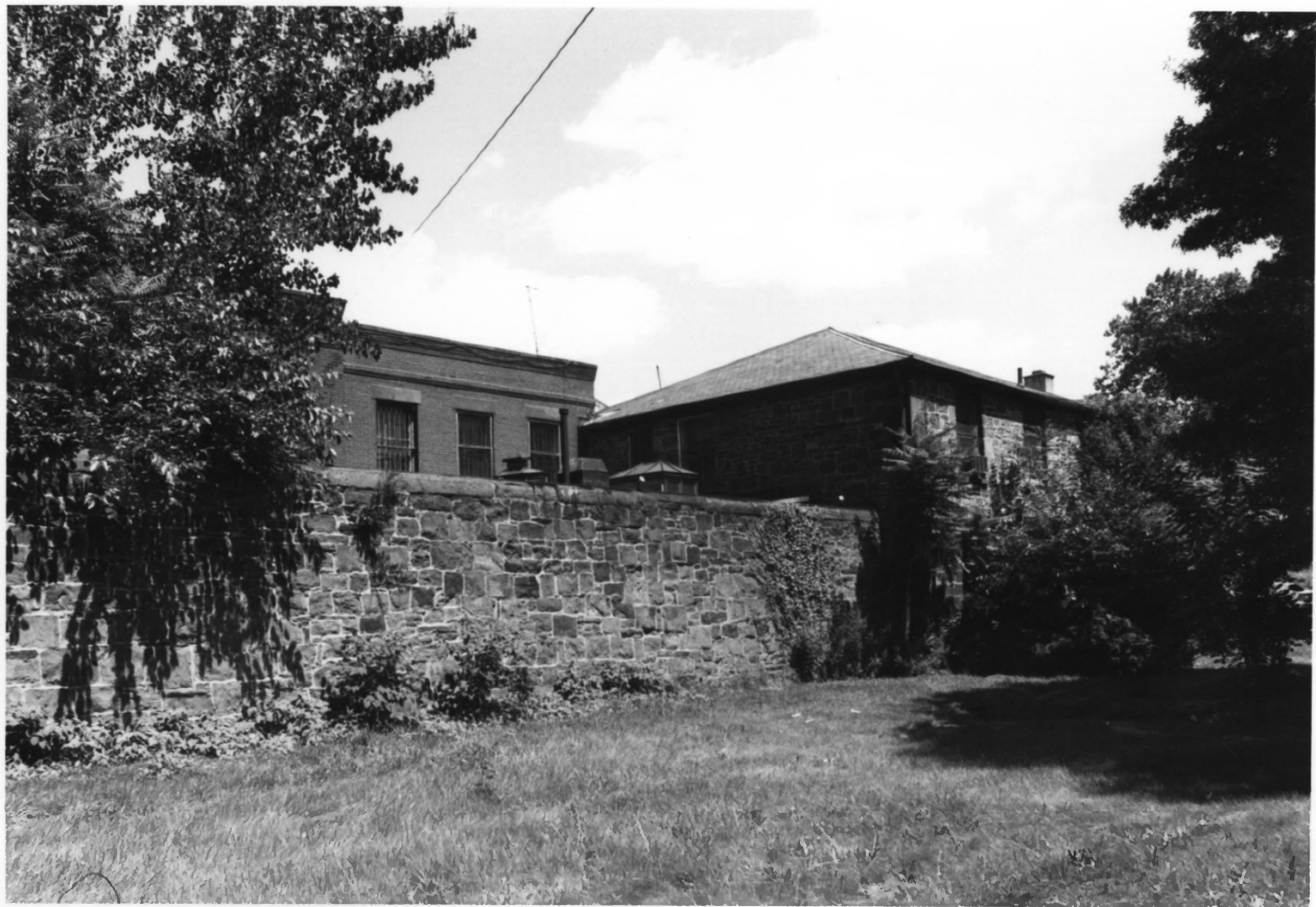
ESSEX COUNTY JAIL NJ ESSEX COUNTY PHOTO 4 OF 9
