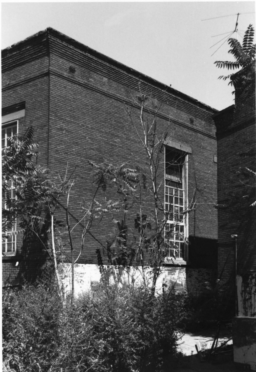
ESSEX COUNTY JAIL NJ ESSEX COUNTY PHOTO 5 OF 9
