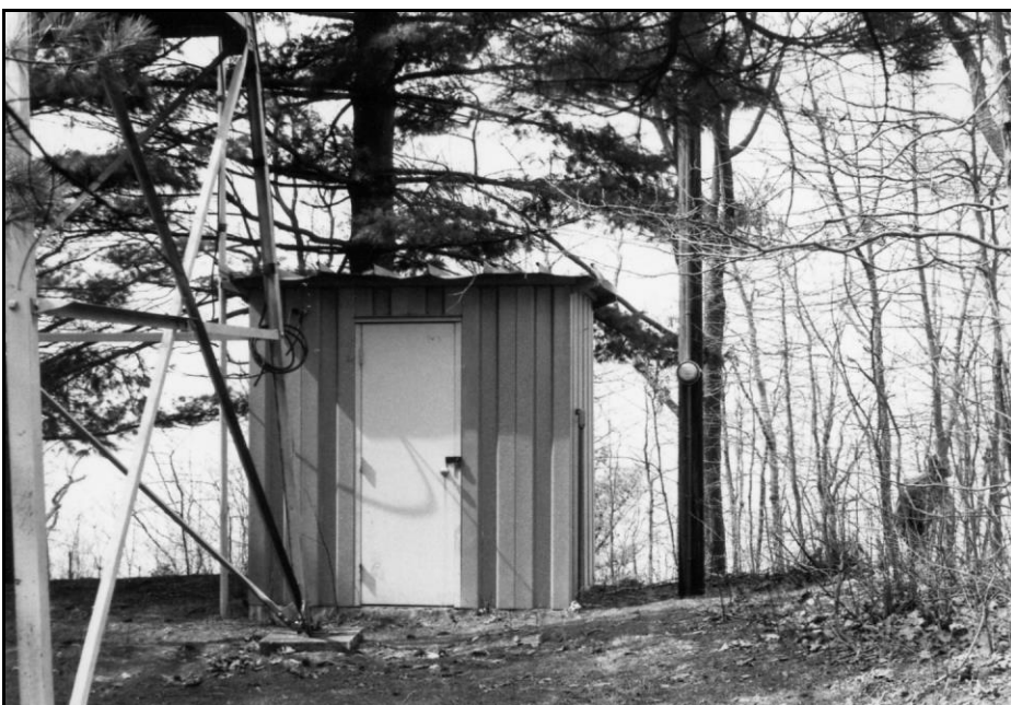
Figure 7: Ca. 1985 photograph of the storage shed (original generator shed) beneath and adjacent to the fire tower; view to the northwest. Photo courtesy of the TN Division of Forestry-East Tennessee District.
