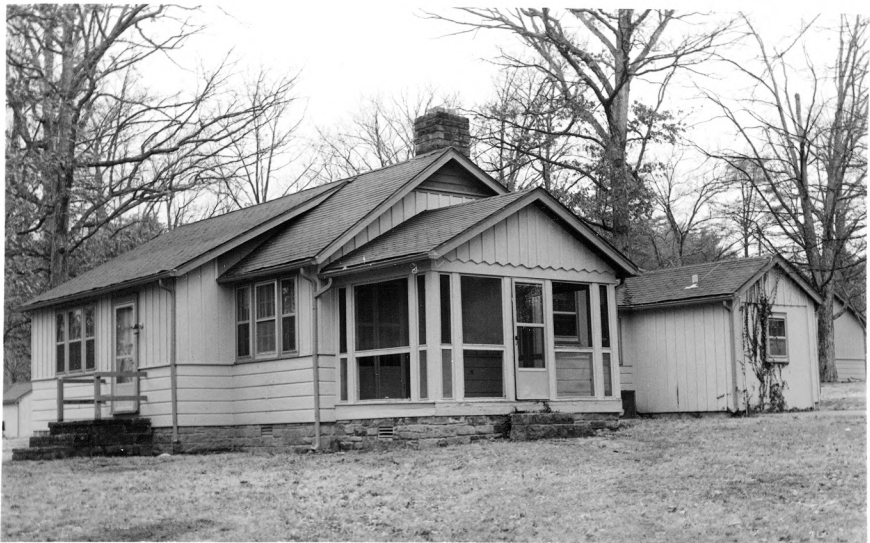
4. Quarters #33, Residential Area District Mammoth Cave National Park, Kentucky
