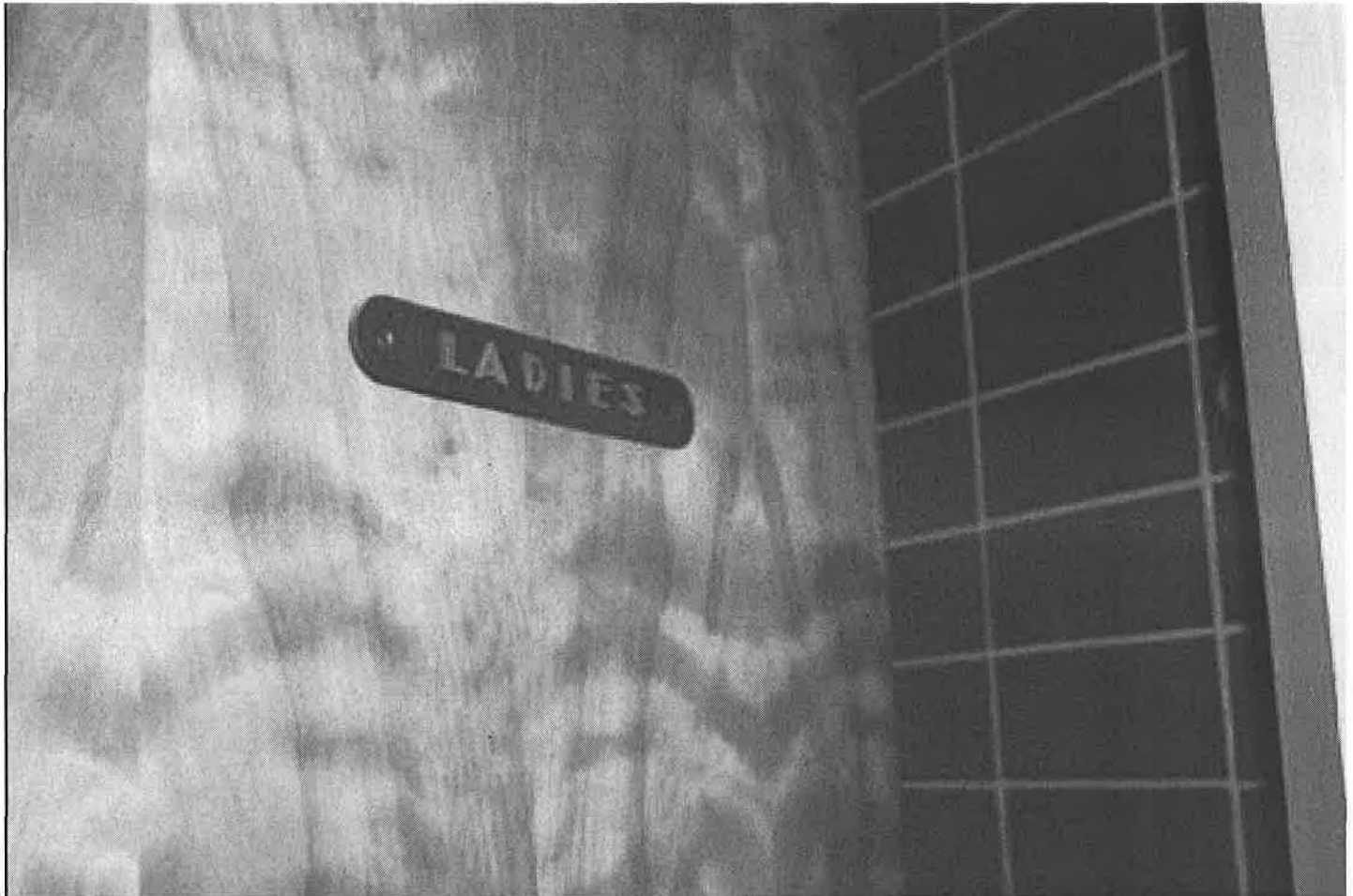
First floor, women's bathroom, view of birch veneer door with "Ladies" name plate and red structural glazed tile.
