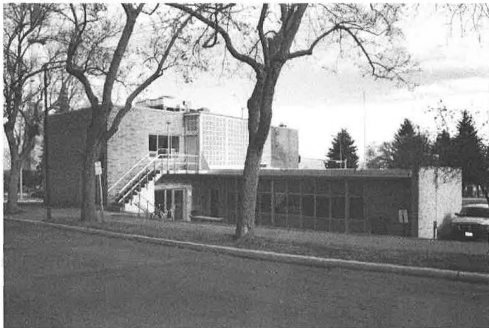
Photo 0002: West and south facades, facing northeast.
