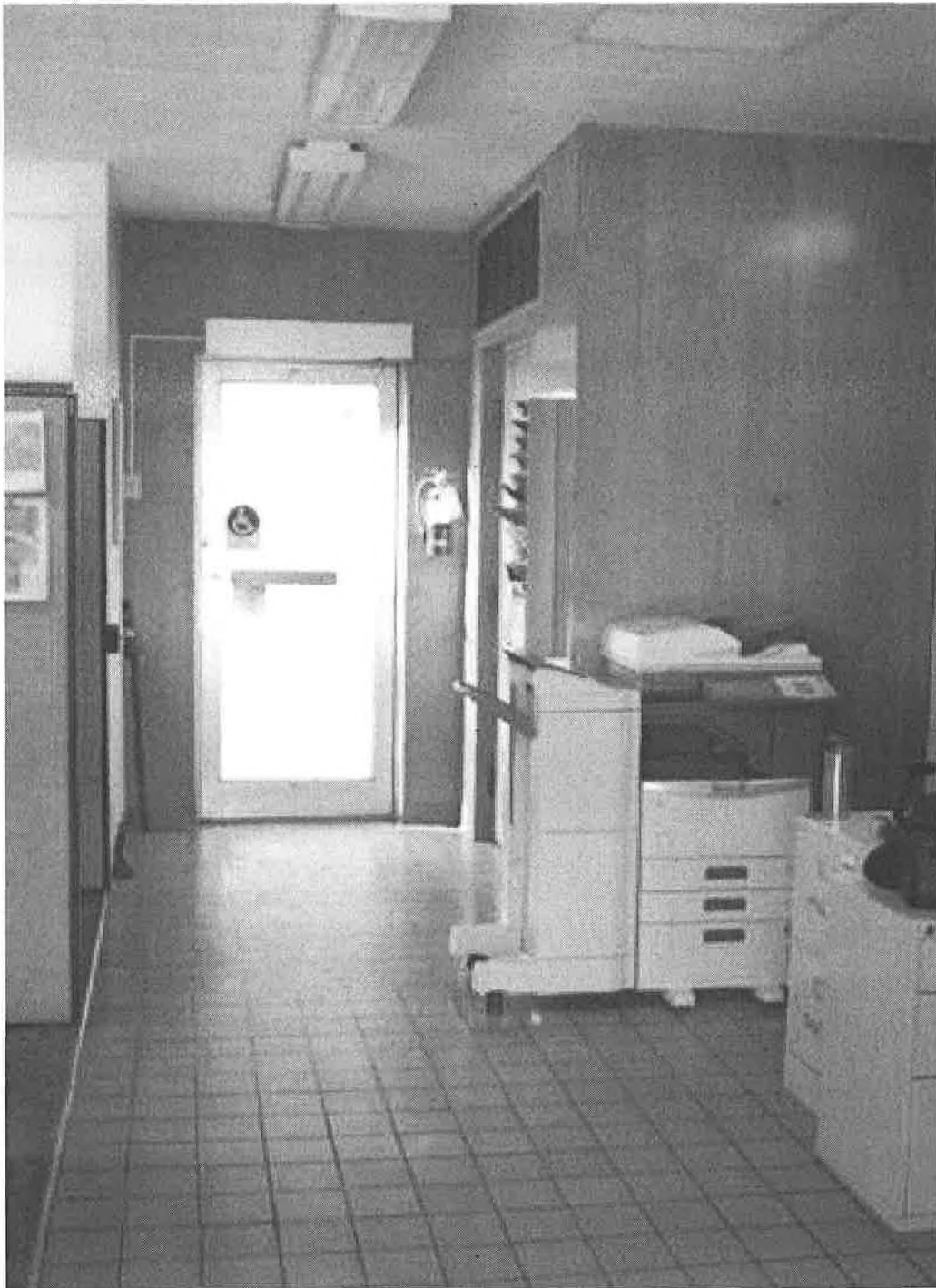
First floor, view of lobby hall with quarry tile floor and rear exit.
