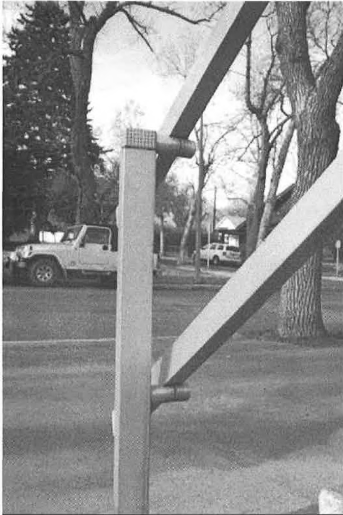
Photo 0011: Stair railing detail, west façade.
