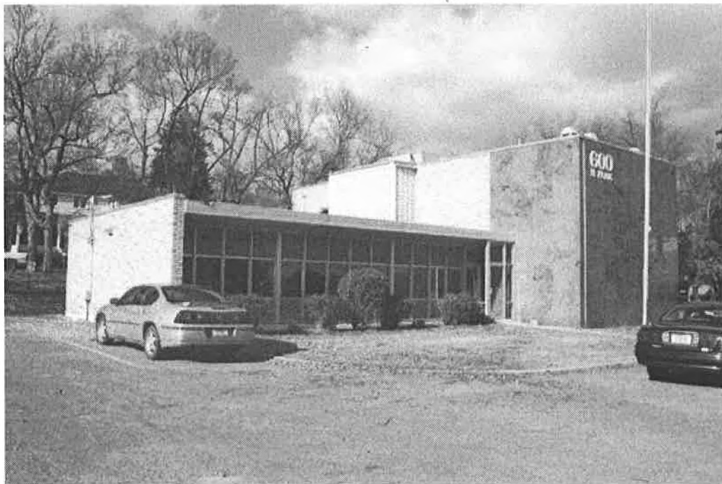
Photo 0001: South and east facades, facing northwest.
