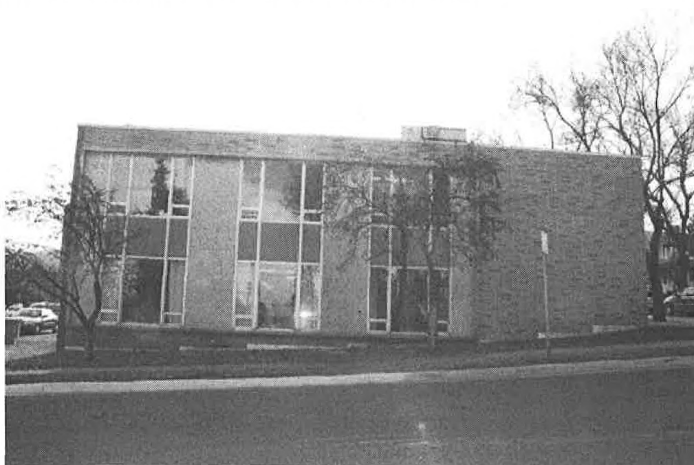
Photo 0003: North façade, facing south.
