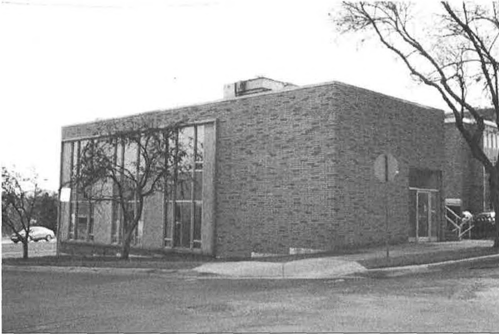
Photo0004: North and west (north end) facades; facing southeast.
