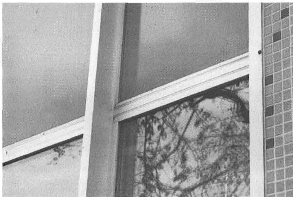
Photo 0009: Curtain wall detail, north façade near center.
