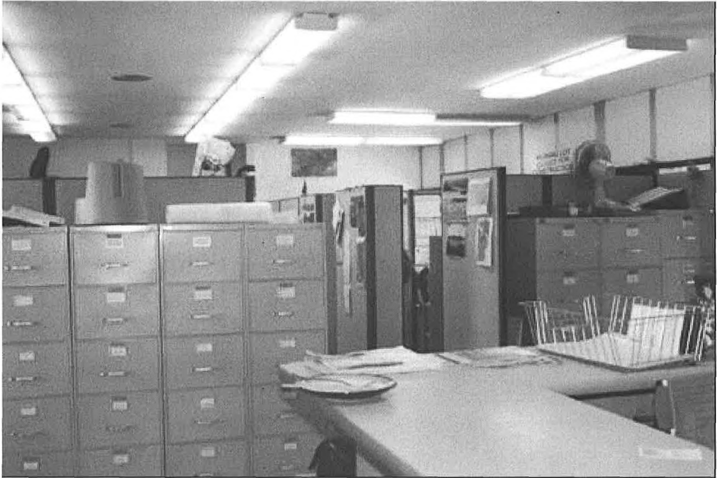
First floor, view of south wing. This wing formerly contained offices for two agents and a superintendent on the west wall, and on the east wall was a large waiting area, another agent office, and a supply room.
