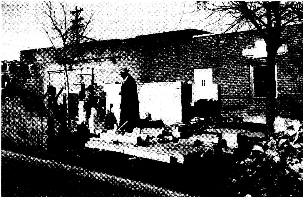
Photo 12. Mount Zion Rebuilding and Integrating Old Church, 1945. 44
