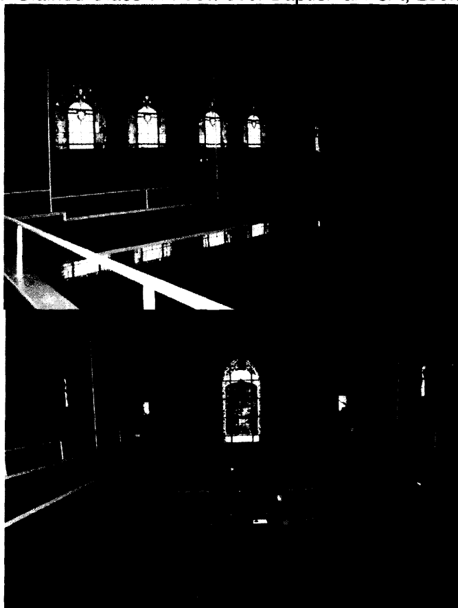
Photos 0006 and 0007. Side Balcony, and Pulpit from the Rear Balcony, Looking North, North East and North East
