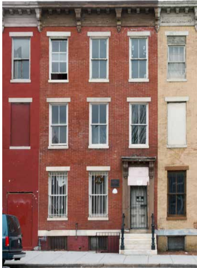
1438 9th St., N.W., Washington, D.C., the former home of Dr. Woodson and headquarters of ASNLH and Associated Publishers, in 2005. NPS Photo
