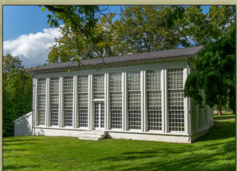
Orangery This modern orangery replaced the original Greek Revival structure, which burned in 1926. The orangery housed citrus fruit trees in the winter, providing fruit throughout the year.
