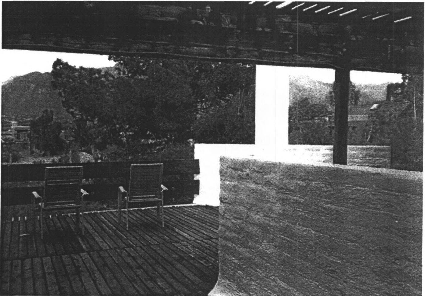
PHOTO 4: Exterior view from roof deck directly under ramada, looking north (Neg. # MAPP-1-24)
