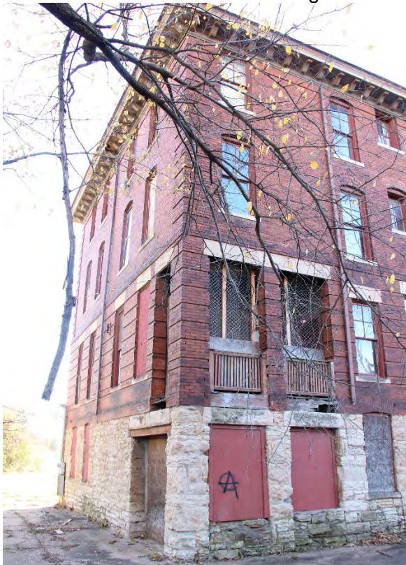
11 of 25: Back wall. Camera facing south.
