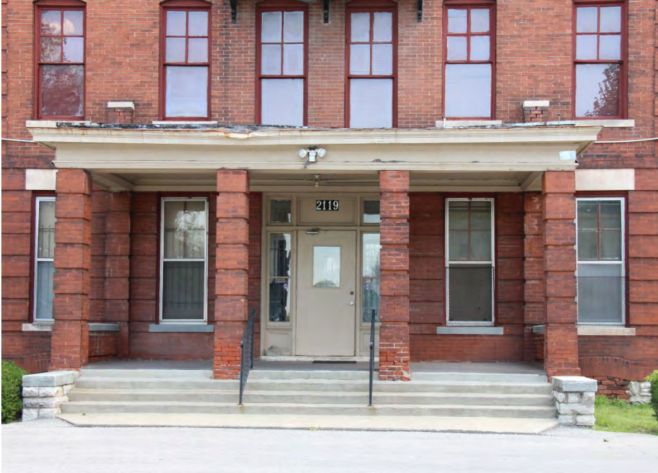
15 of 25: Front porch with main entry. Camera facing east.
