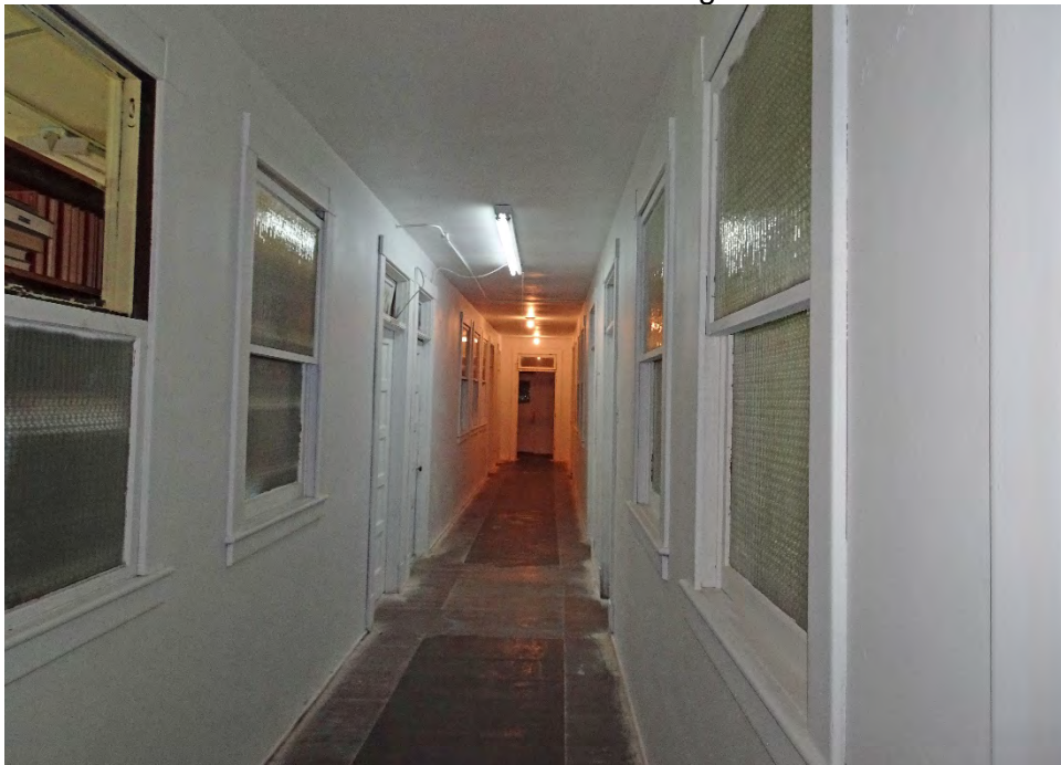
19 of 25: Second floor central hall. Camera facing west.
