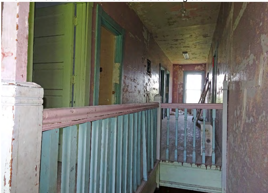
22 of 25: Back hall of third floor. Camera facing south.
