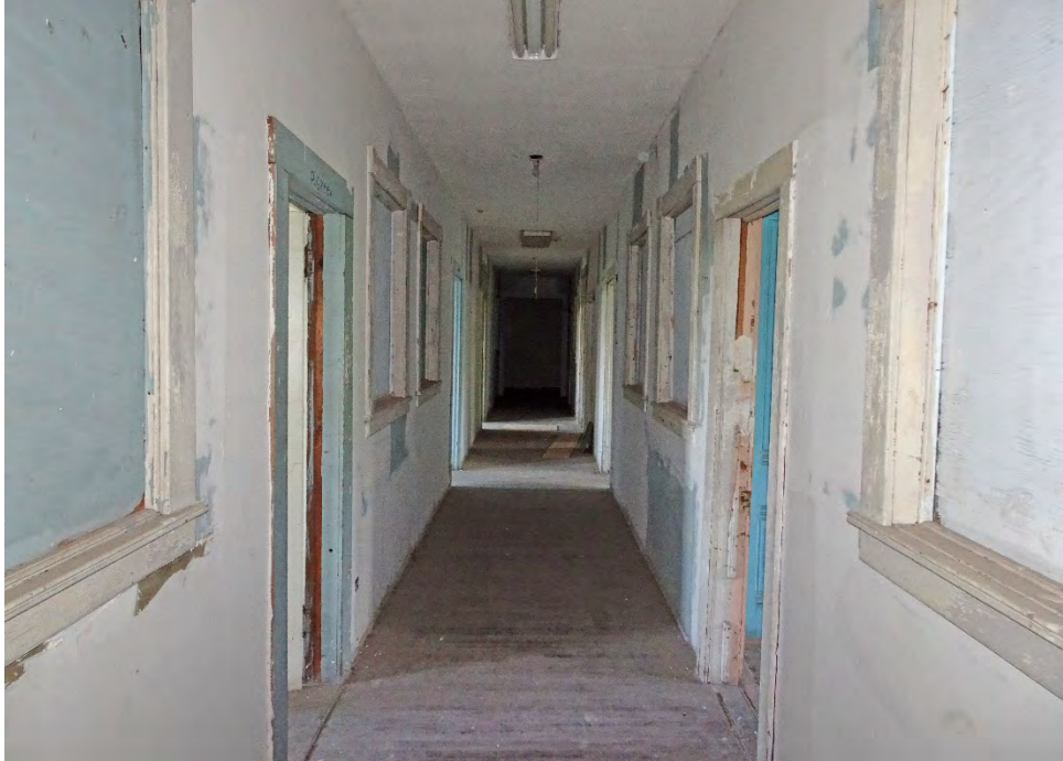
25 of 25: Third floor central hall. Camera facing east.
