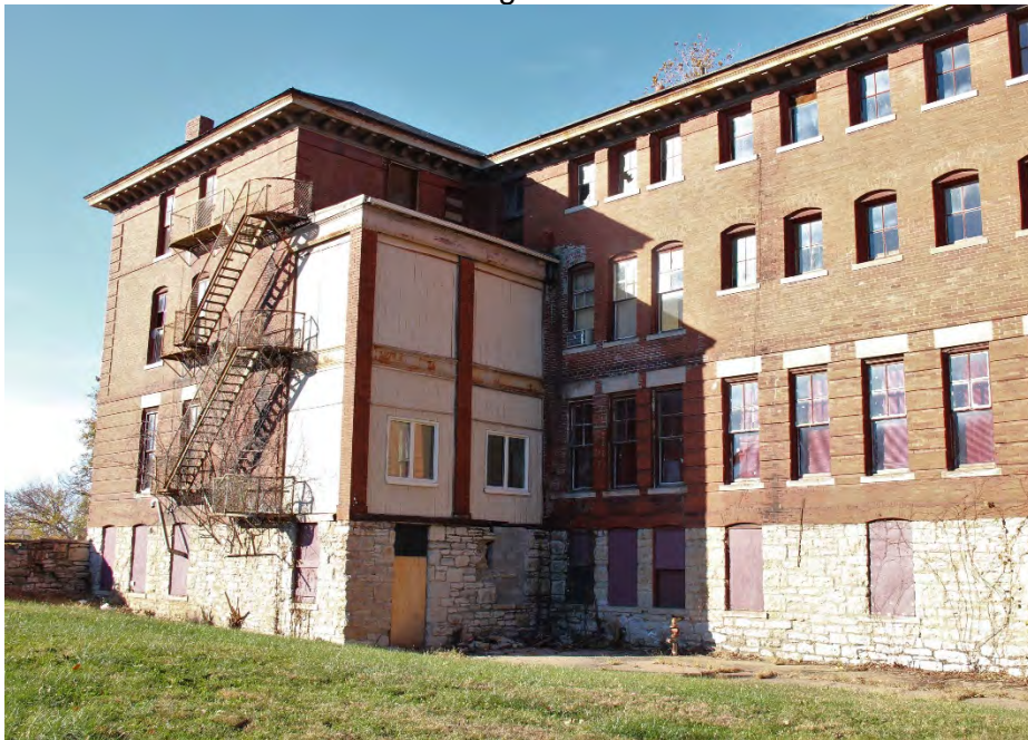
9 of 25: South side. Camera facing northwest.
