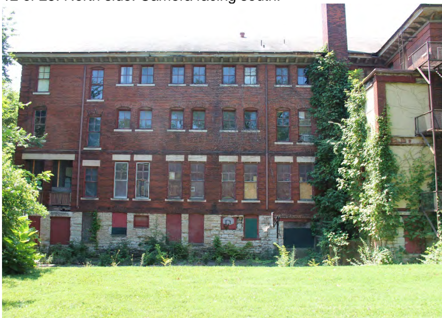
12 of 25: North side. Camera facing south.
