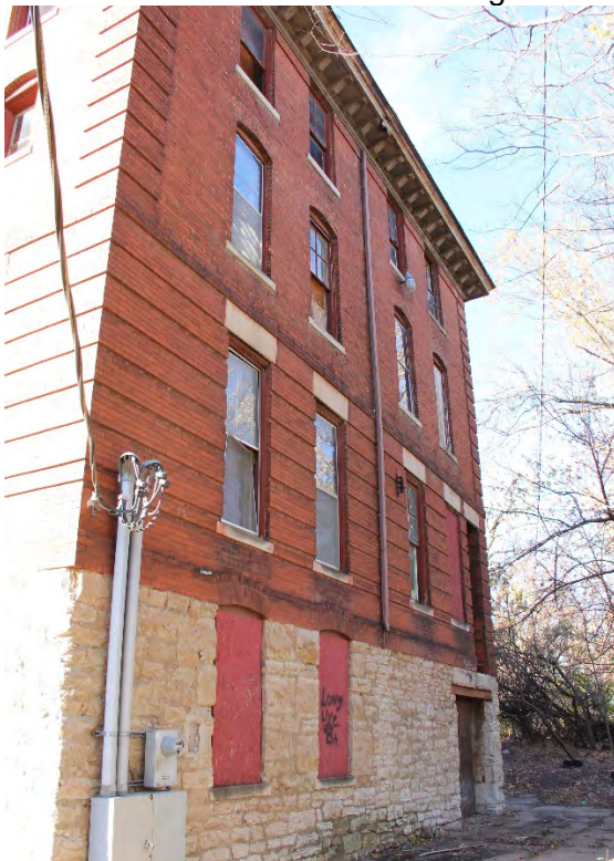
10 of 25: Back wall. Camera facing northwest.
