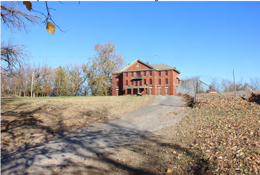
5 of 25: Façade from circle drive. Camera facing east.
