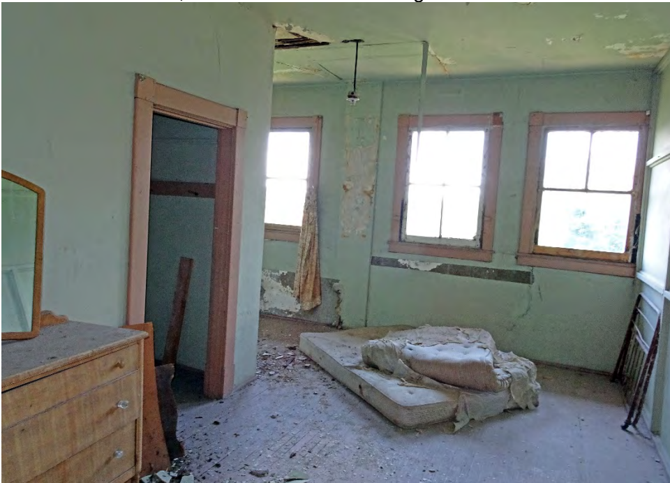
24 of 25: Third floor, rear block. Camera facing south.
