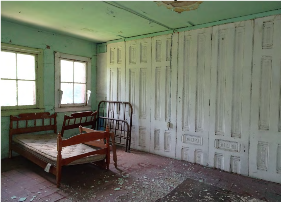
23 of 25: Third floor, rear block. Camera facing northeast.
