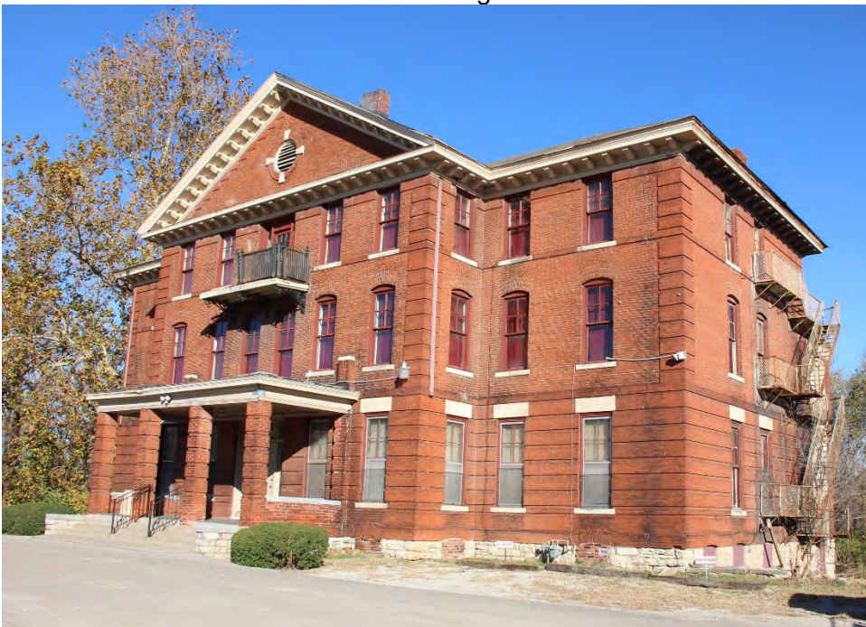
6 of 25: Southwest corner. Camera facing northeast.
