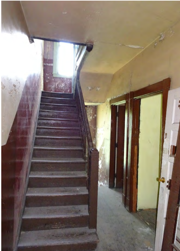
21 of 25: Back staircase to second floor. Camera facing north.
