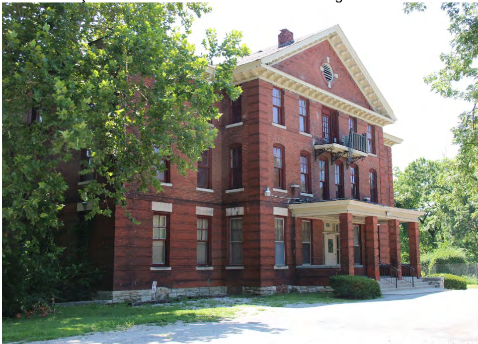
14 of 25: Façade at northwest corner. Camera facing southeast.
