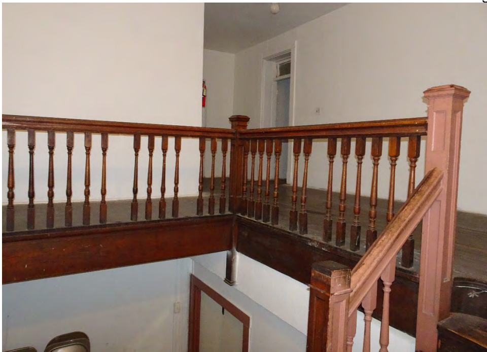
18 of 25: Second floor north-south hall with main staircase. Camera facing northeast.
