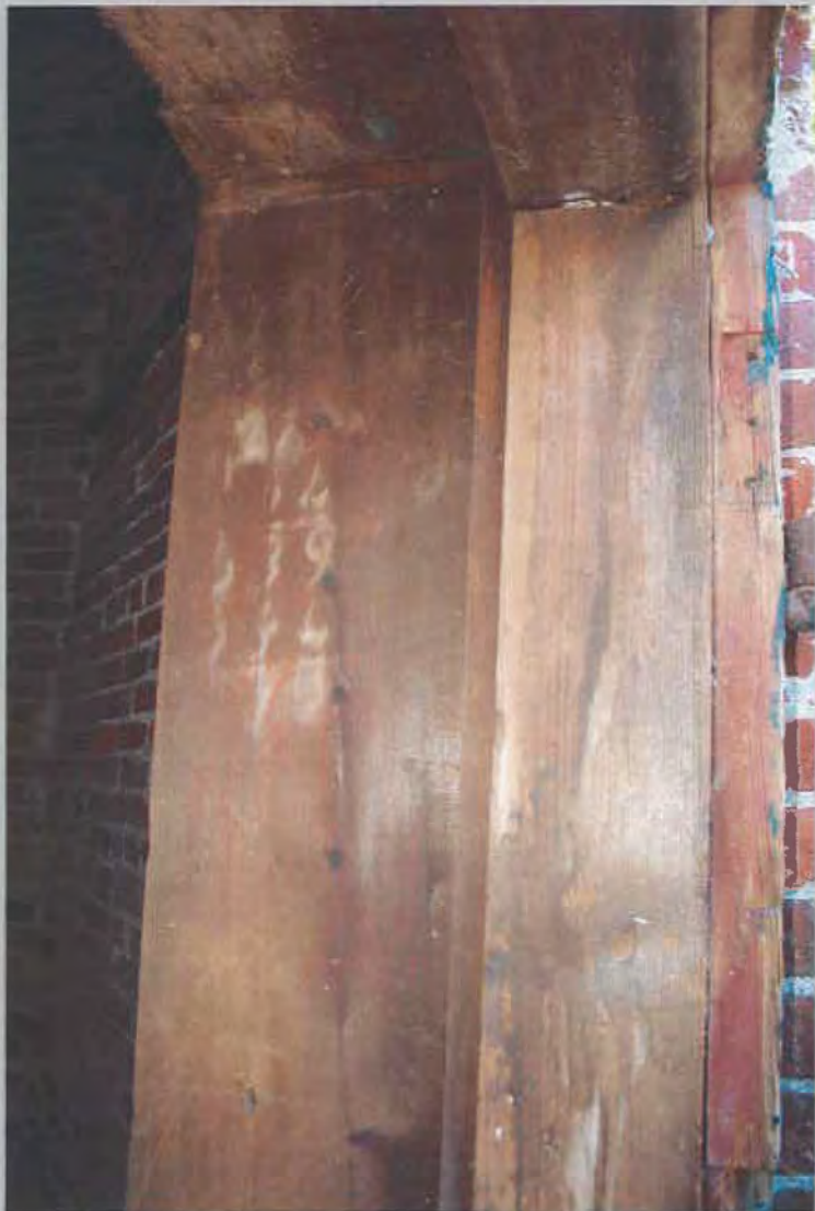
7. Right (south) side of door frame. View SE.
