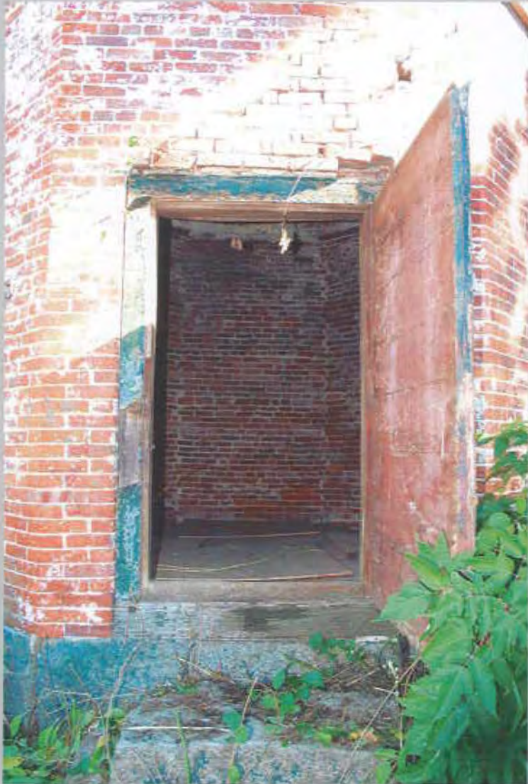
5. Entry opening to interior chamber. View NE.
