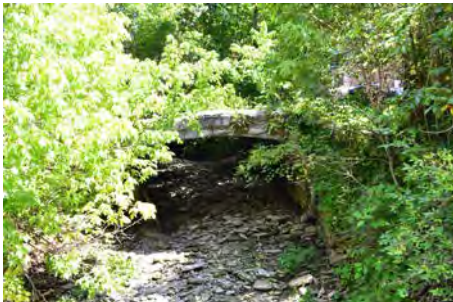
West Concrete Reinforced Bridge (27)
