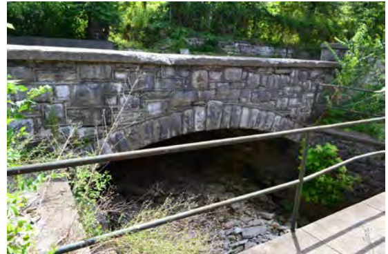
Cut Stone Bridge (25)
