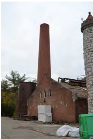
Boiler Room (Feature 3)
