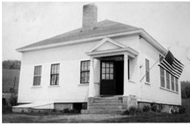
Root School, Norwich, Windsor Co., Vermont Photograph #3 of 15 Root School, undated historic view c. 1940, looking northwest (Courtesy Norwich Historical Society)
