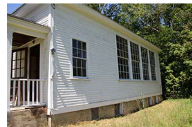
Root School, Norwich, Windsor Co., Vermont Photograph #9 of 15 Root School east elevation, view looking northwest
