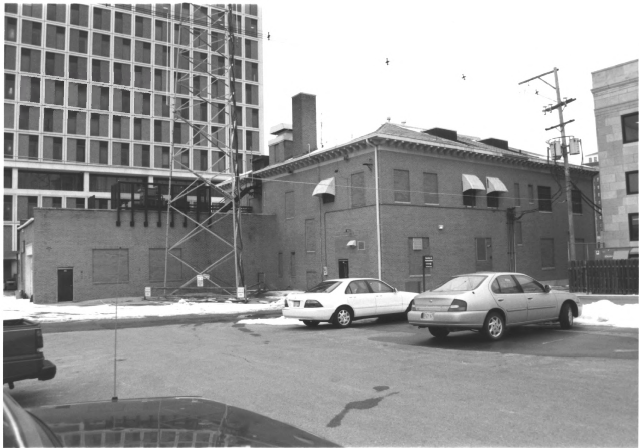
TOPEKA FIRE STATION #2, SHAWNEE COUNTY, KANSAS #5
