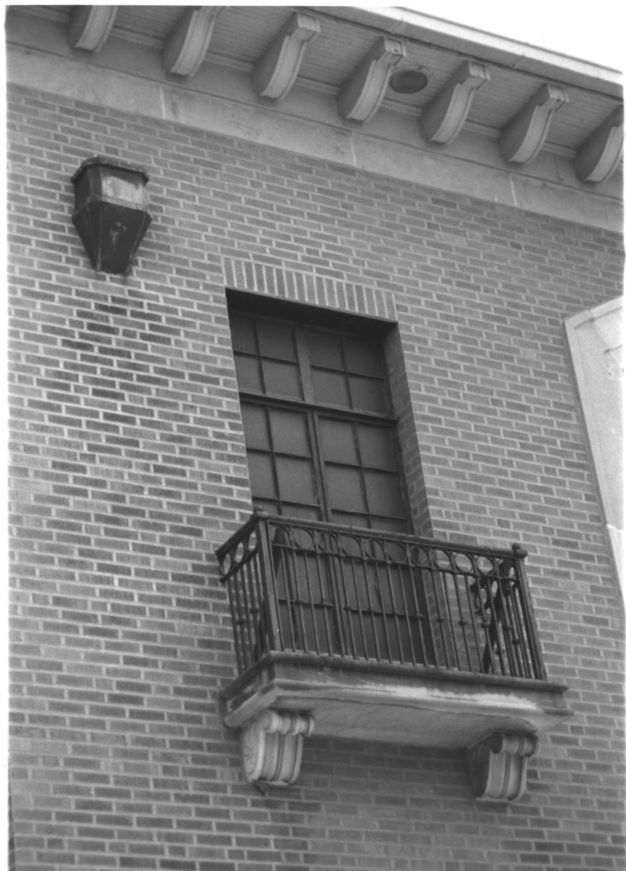
TOPEKA FIRE STATION #2, SHAWNEE COUNTY, KANSAS #6
