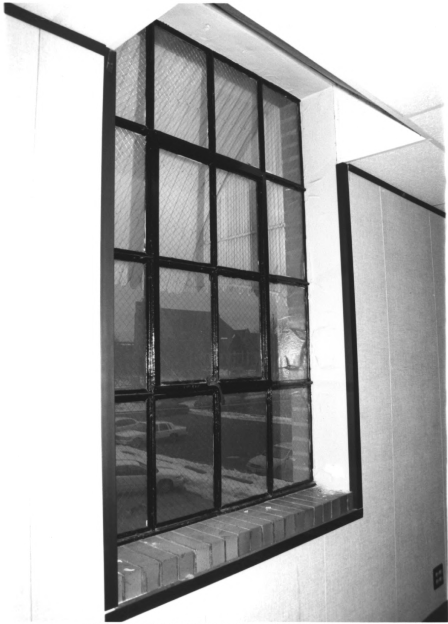
TOPEKA FIRE STATION #2, SHAWNEE COUNTY, KANSAS #23
