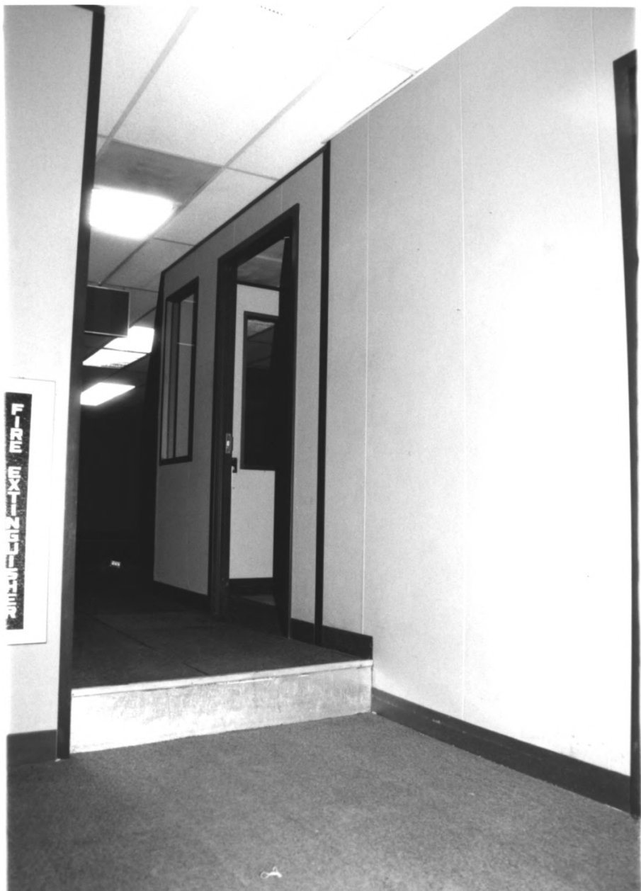
TOPEKA FIRE STATION #2, SHAWNEE COUNTY, KANSAS #21
