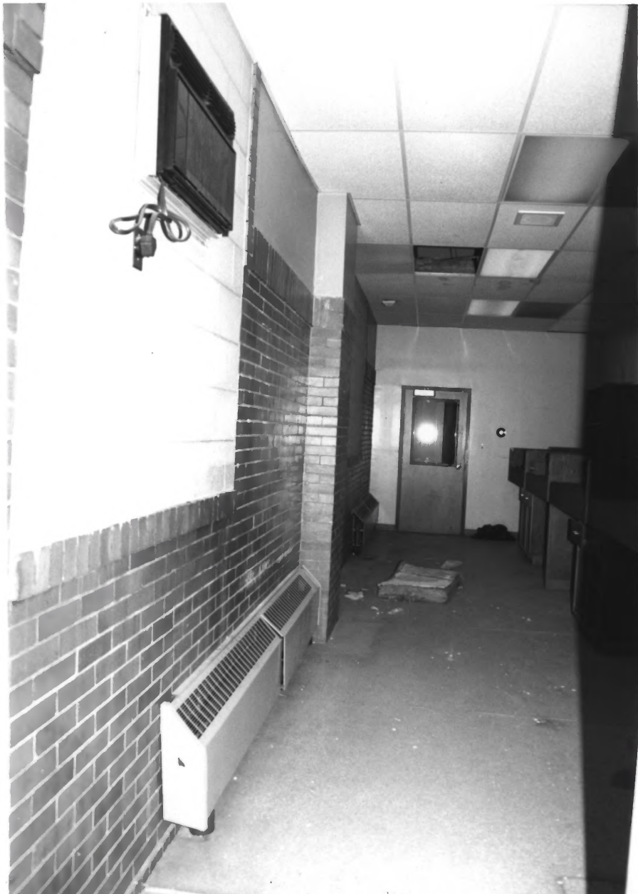
TOPEKA FIRE STATION #2, SHAWNEE COUNTY, KANSAS #14
