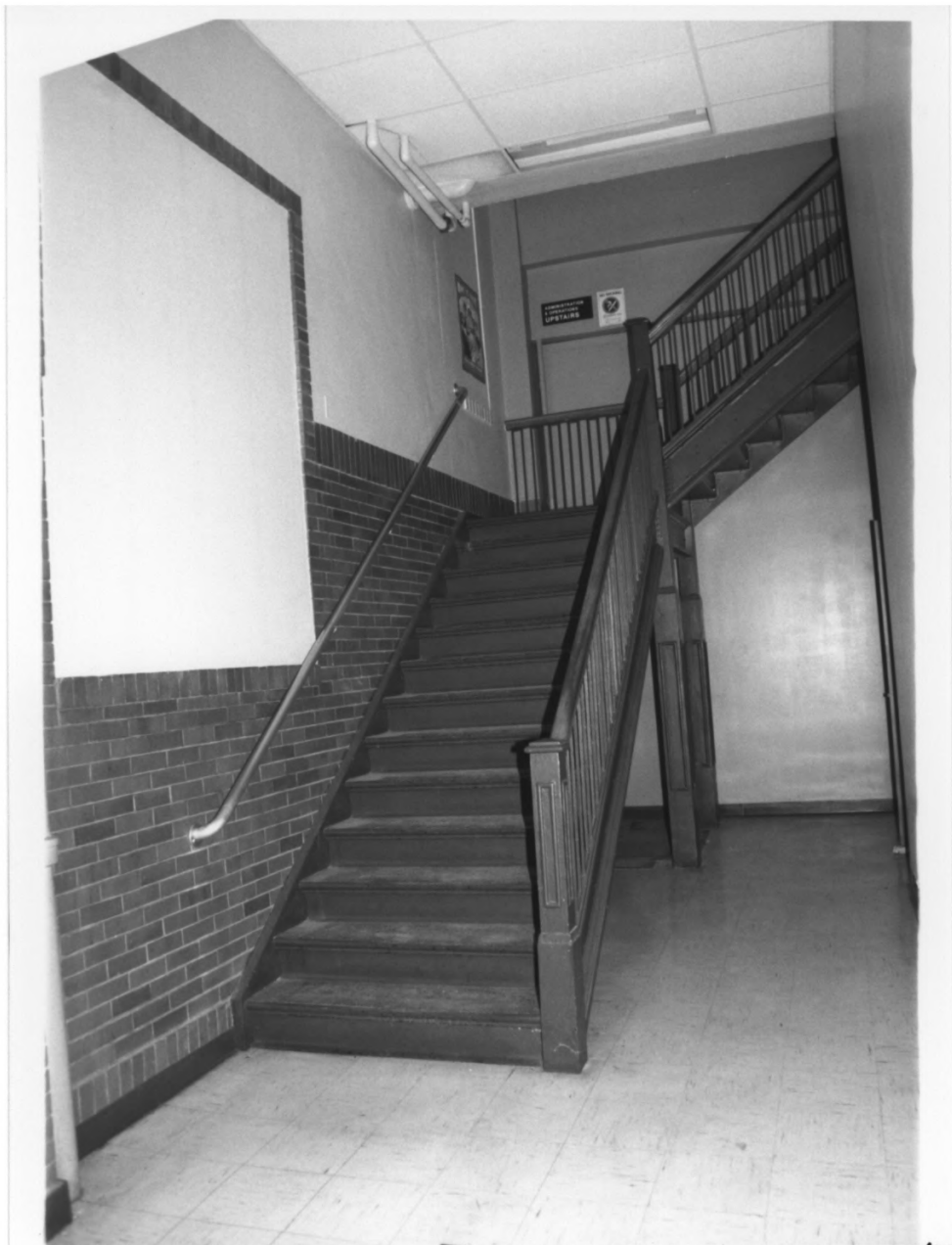
TOPEKA FIRE STATION #2, SHAWNEE COUNTY, KANSAS #17
