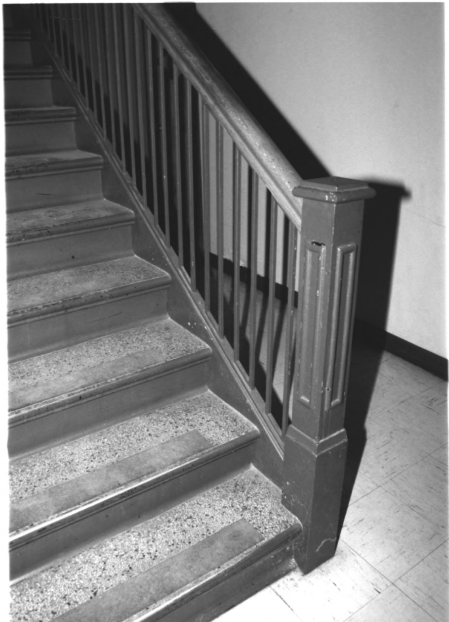
TOPEKA FIRE STATION #2 . SHAWNEE COUNTY, KANSAS #18
