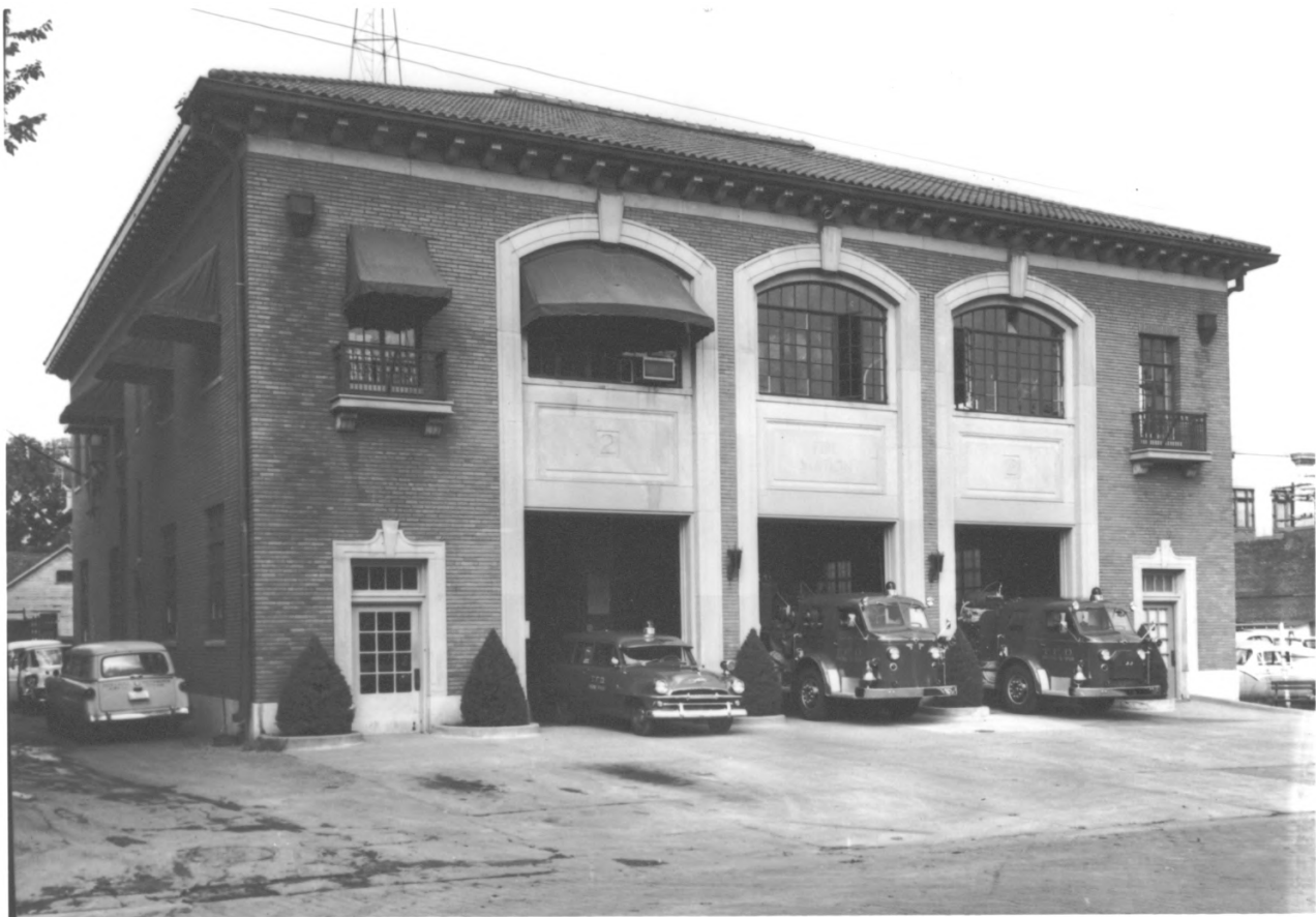
TOPEKA FIRE STATION #2, SHAWNEE COUNTY, KANSAS #25
