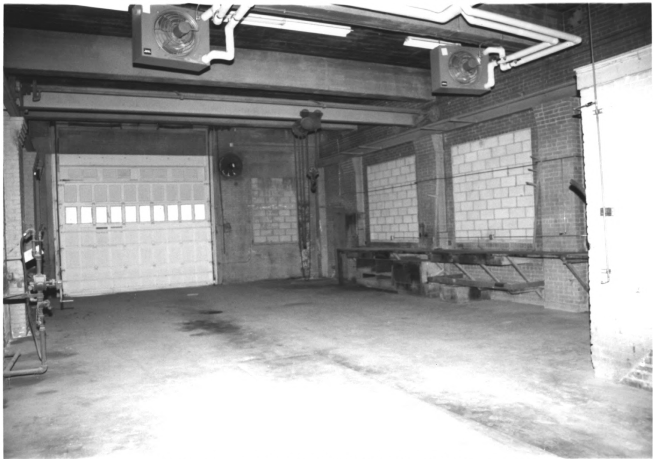
TOPEKA FIRE STATION #2, SHAWNEE COUNTY, KANSAS #10
