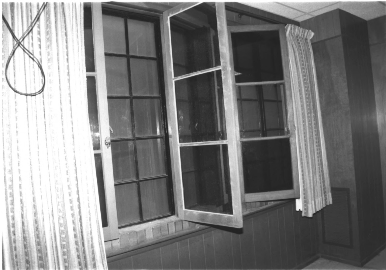
TOPEKA FIRE STATION #2, SHAWNEE COUNTY, KANSAS #2A
