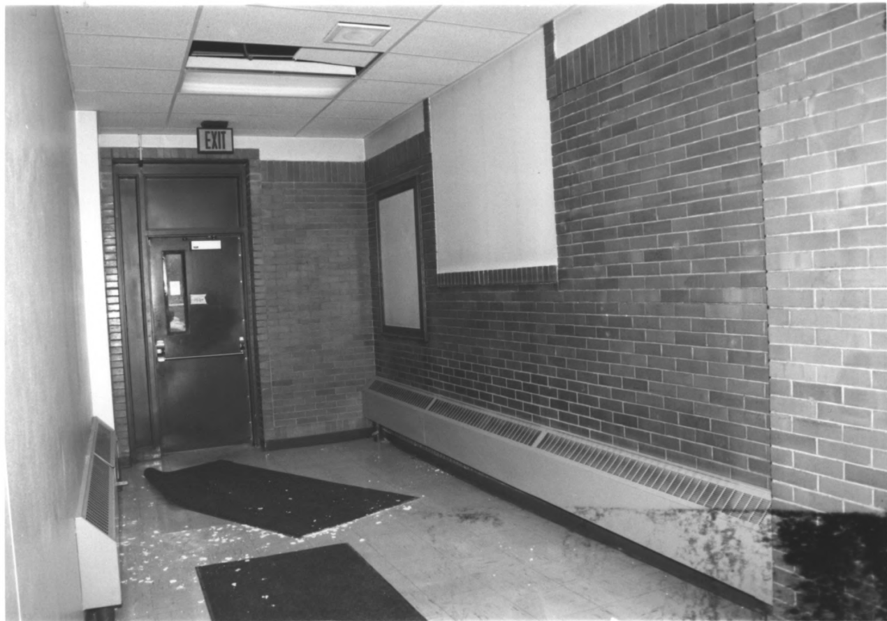
TOPEKA FIRE STATION #2, SHAWNEE COUNTY, KANSAS
