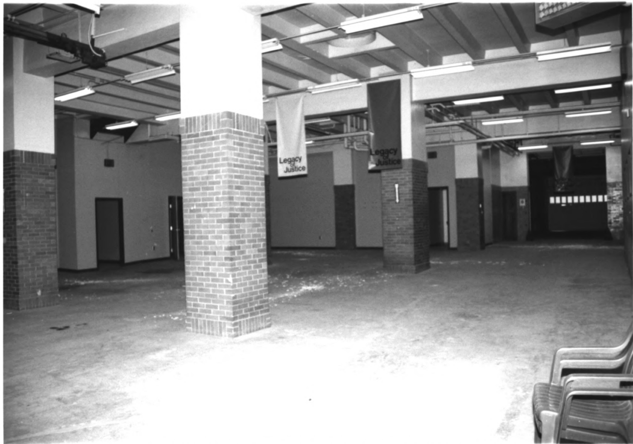
TOPEKA FIRE STATION #2, SHAWNEE COUNTY, KANSAS #9
