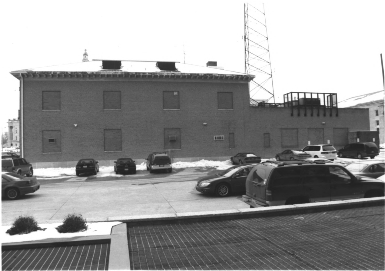
TOPEKA FIRE STATION #2, SHAWNEE COUNTY, KANSAS
