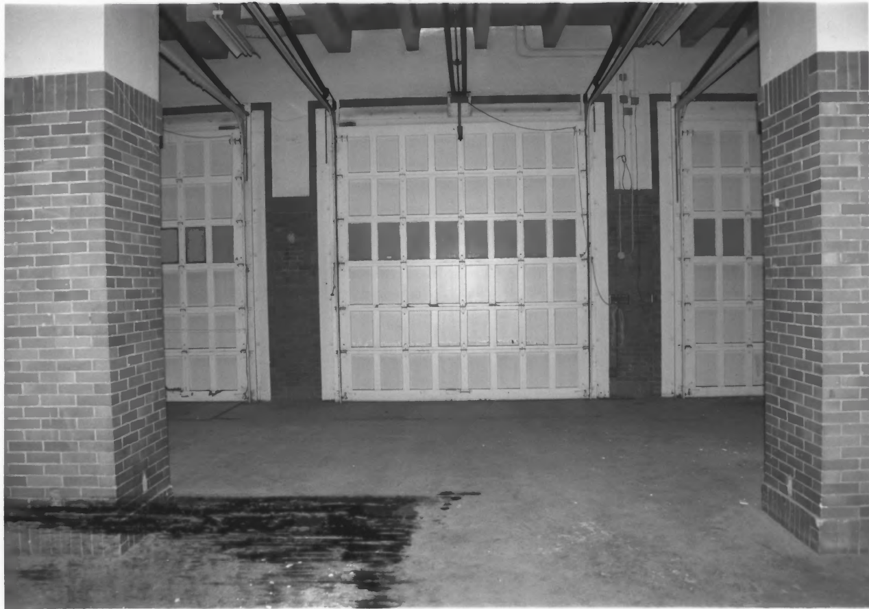
TOPEKA FIRE STATION #2, SHAWNEE COUNTY, KANSAS
