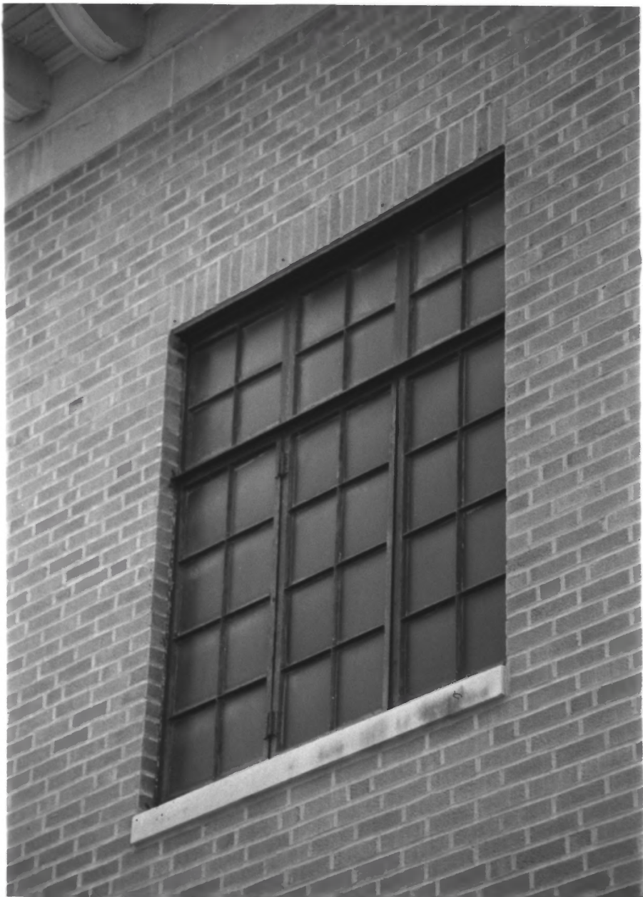
TOPEKA FIRE STATION #2, SHAWNEE COUNTY, KANSAS #7
