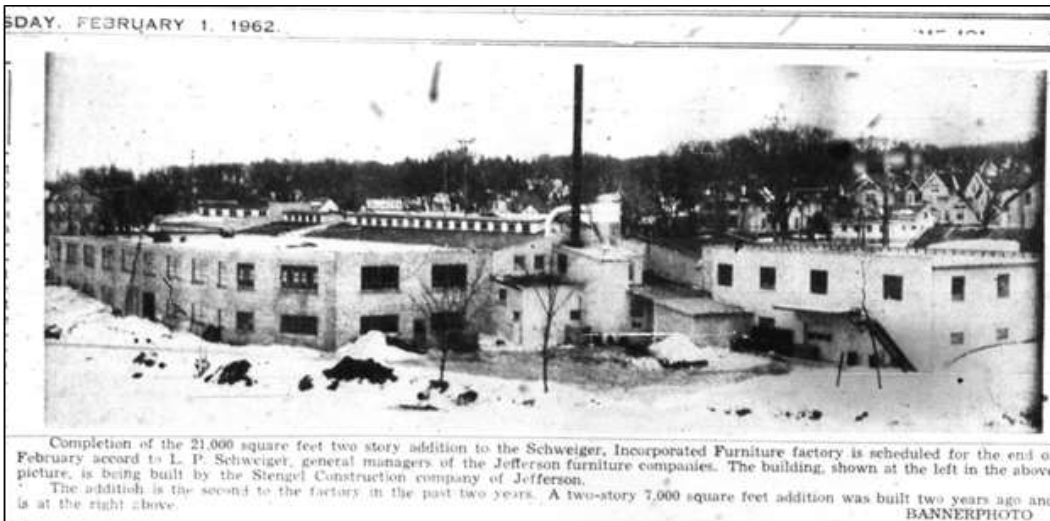
Figure 4: Schweiger Industries Plant III in 1962 with new two-story addition on left, looking northeast.
