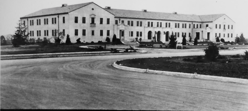
SV-100214 - 1 February 1974, Contract NOy 1873 Specification #7255 Landscaping - View Looking South Toward Bachelor Officers' Quarters
