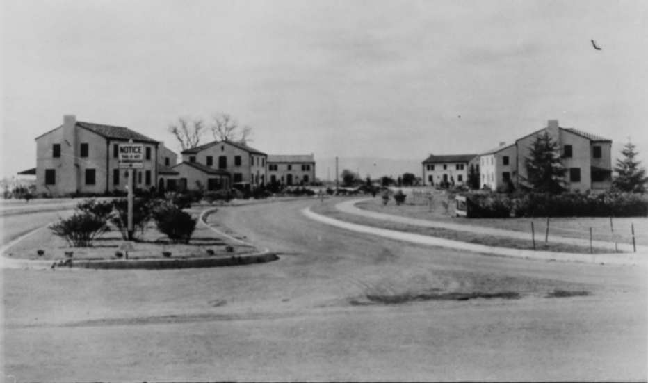
SV-100282 - 1 April 1934. Contract W0Y 1473 Specification 7255 Landscaping - General View of Officers' Quarters Looking South from Clark Road
