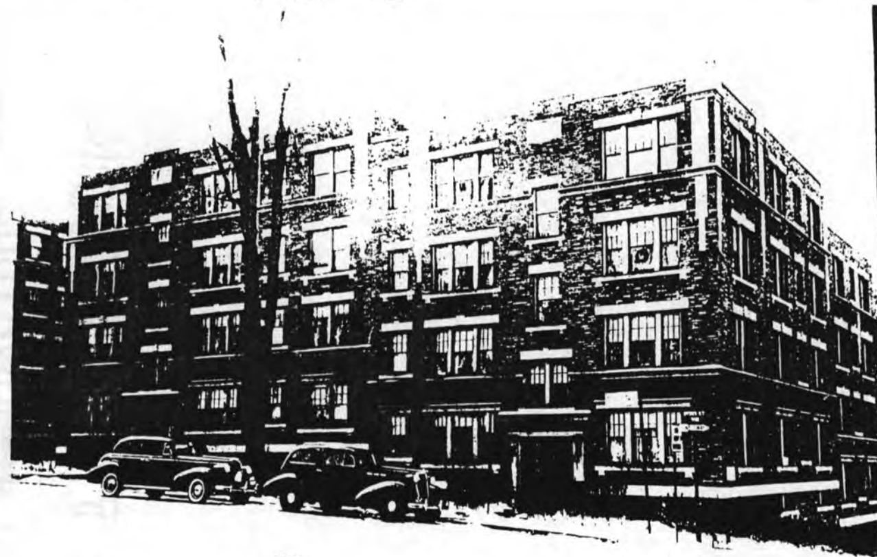
124 - 130 Byers Street, c. 1940 Springfield, MA, Building Department Photograph
