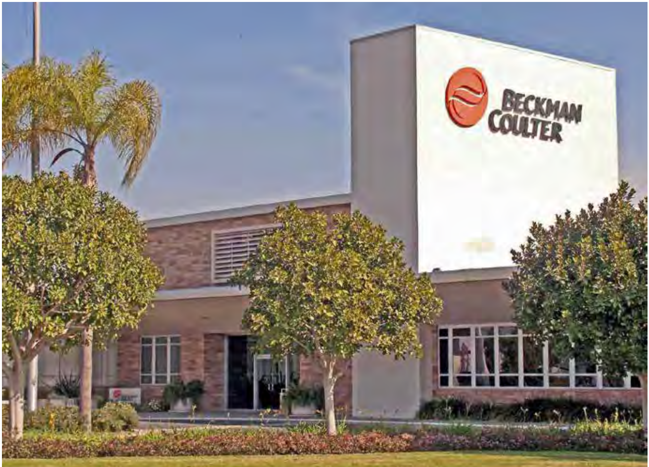
Figure 16: Partial west elevation of building, 2006; camera facing northeastward
