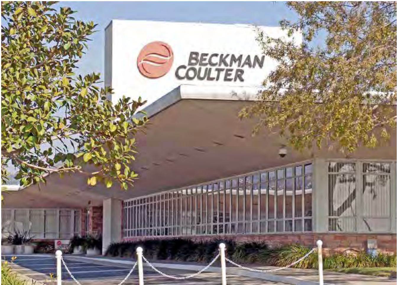
Figure 15: Partial west elevation of building, 2006; camera facing northward from south end of property
