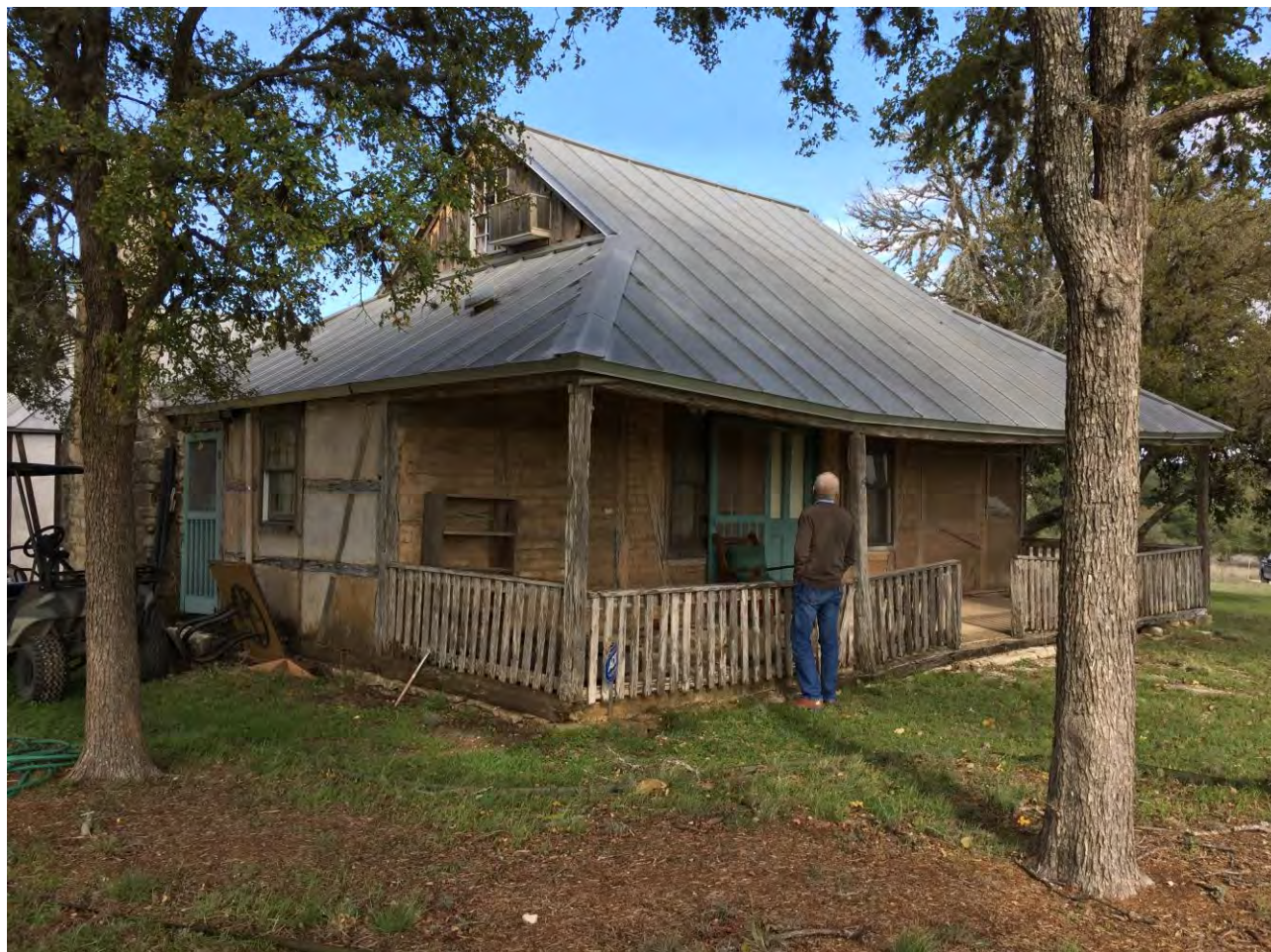
Photo 3 South and west elevations looking northeast David Hannan, November 2015
