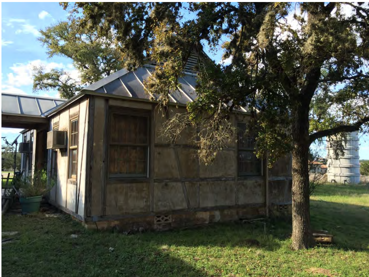
Photo 8 East elevation, non-contributing c. 1980 structure looking northwest David Hannan, October 2016
