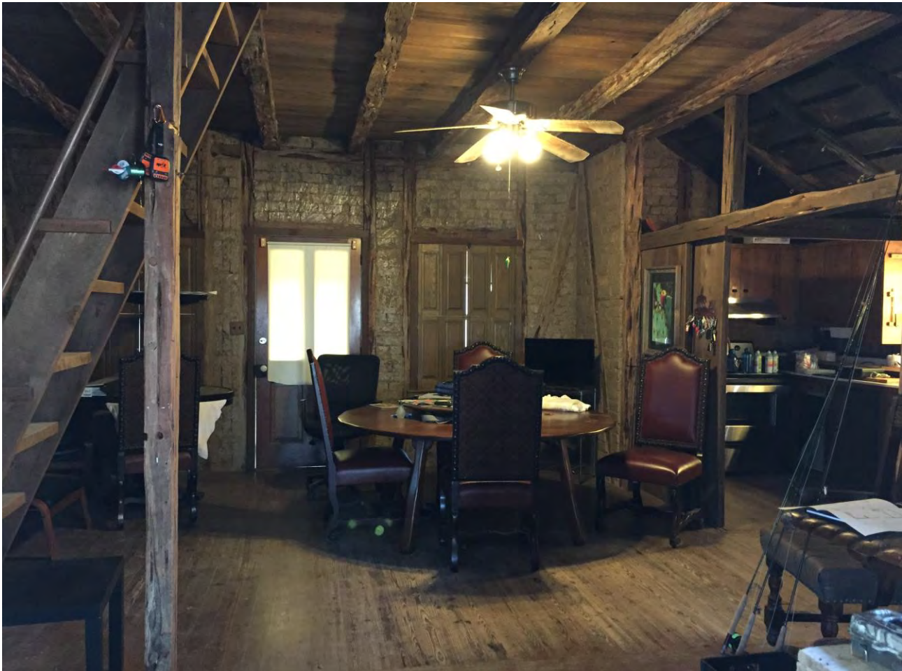
Photo 9 Interior looking south David Hannan, October 2016
