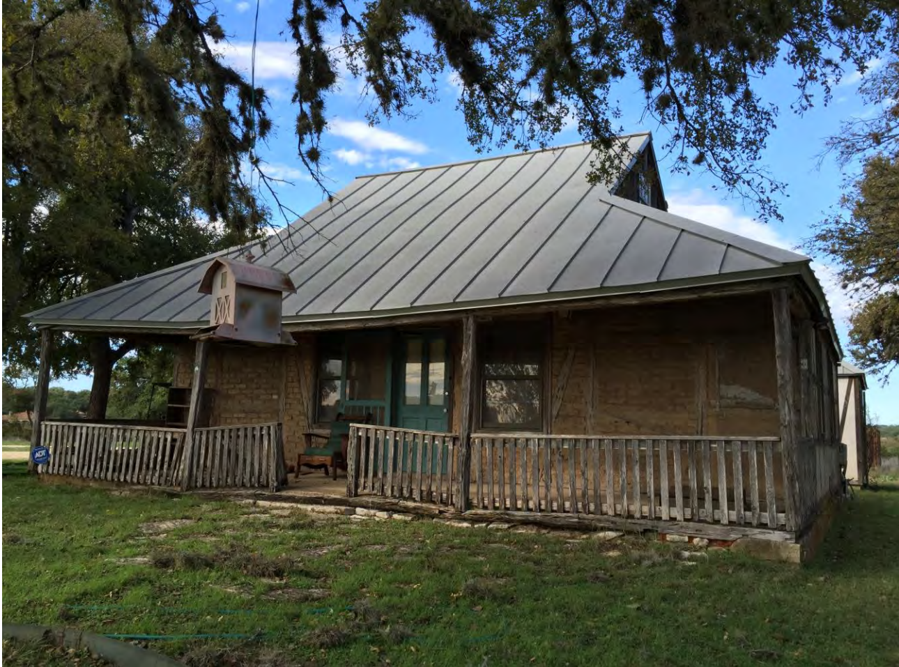
Photo 2 South elevation looking northwest David Hannan, November 2015
