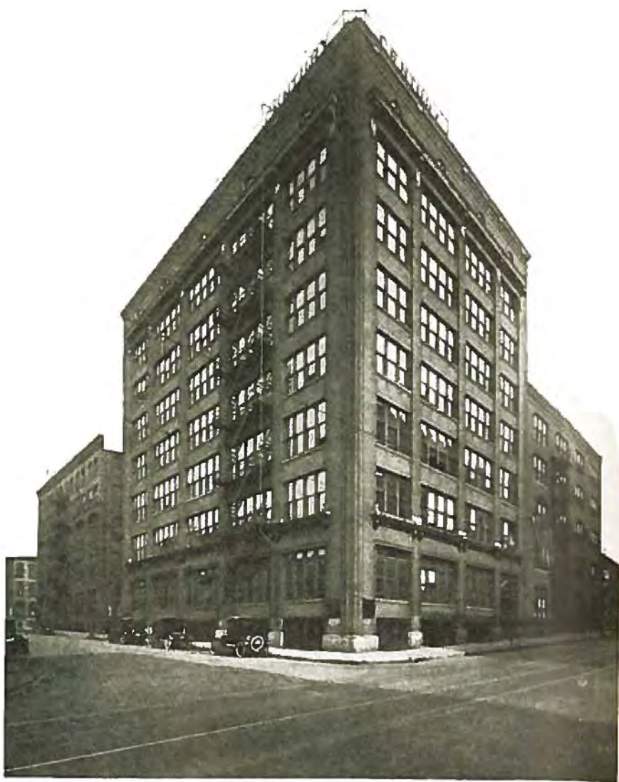
Main plant of the Century Electric Company, the largest manufacturer of single phase motors in St. Louis.
