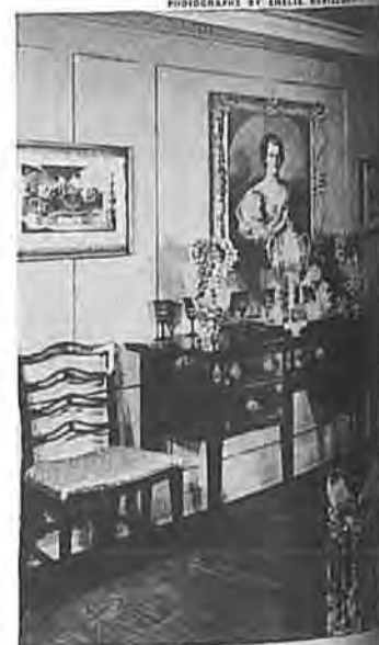
Not only the walls and ceilings in this house are pressed wood, but even the family portraits have been painted on it. Solid wood is used for doors and cabinets since pressed wood is made in sheets not much thicker than 1/4"
