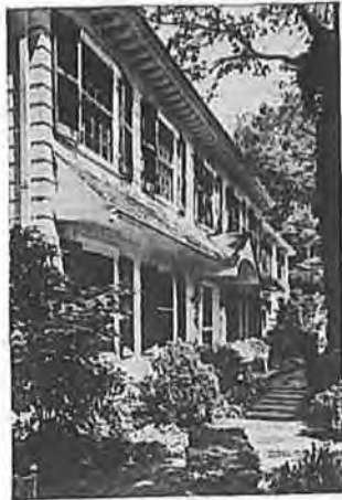
Greenbrier's window and doorway overhangs are lined with pressed wood which was also used as sheathing in the construction of the house. It's moisture-resistant, durable
