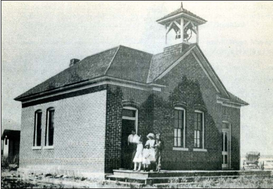
Figure 2. This ca. 1900-03 photograph of the Gas Creek School (view northwest) shows the original 1889-90 building and demonstrates that the same design was followed in the 1909 rebuilding. The image shows a full-width wood deck across the front and a privy at the left edge. Courtesy of Shaputis, Where the Bodies Are in Central Chaffee County, Colorado (1995), 37.
