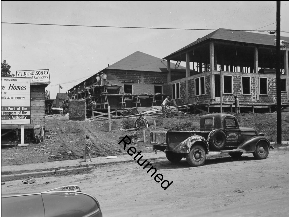
Figure 1. Construction of the James A. Cayce Administration Service Building in 1942. (Metro Nashville Archives)
