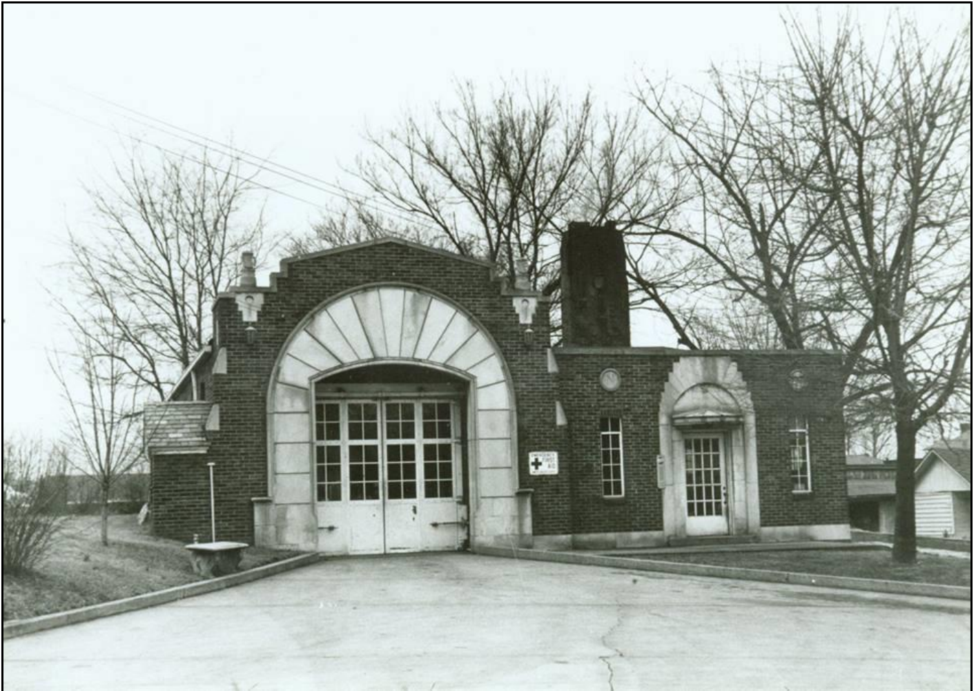
Figure 1: Fire Hall for Engine Company No. 18, date unknown.
