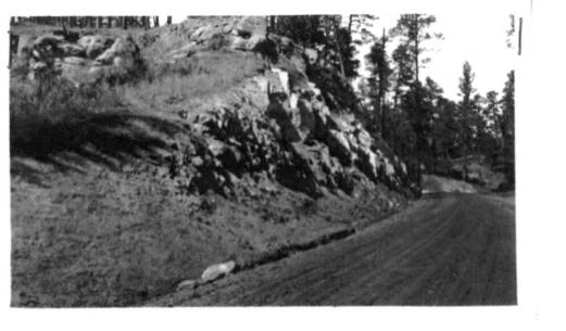
"Showing manner in which rock cut slopes left in rough state."
