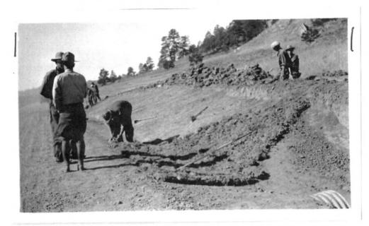
"Resodding ditch line and cut slope after flattening and rounding along entrance highway."
