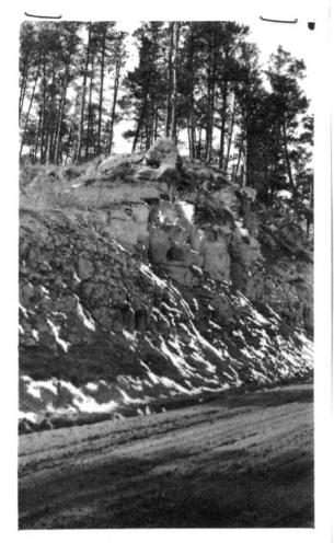
"Roadside cut slope not touched except removal of loose material."
