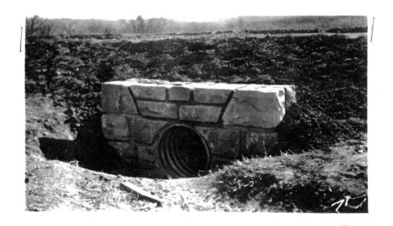
"Showing headwall typical of those constructed along entrance highway"
