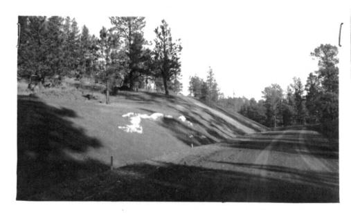
"Showing cut slope after flattening and rounding."
