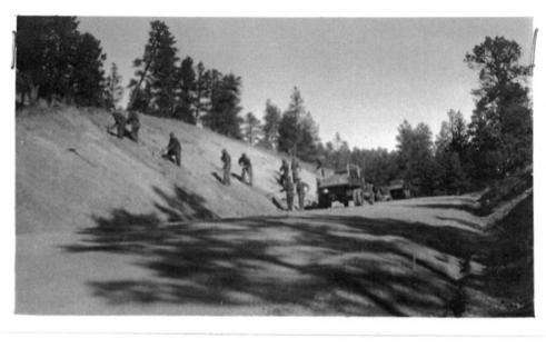
"Flattening and rounding cut slope along entrance highway."
