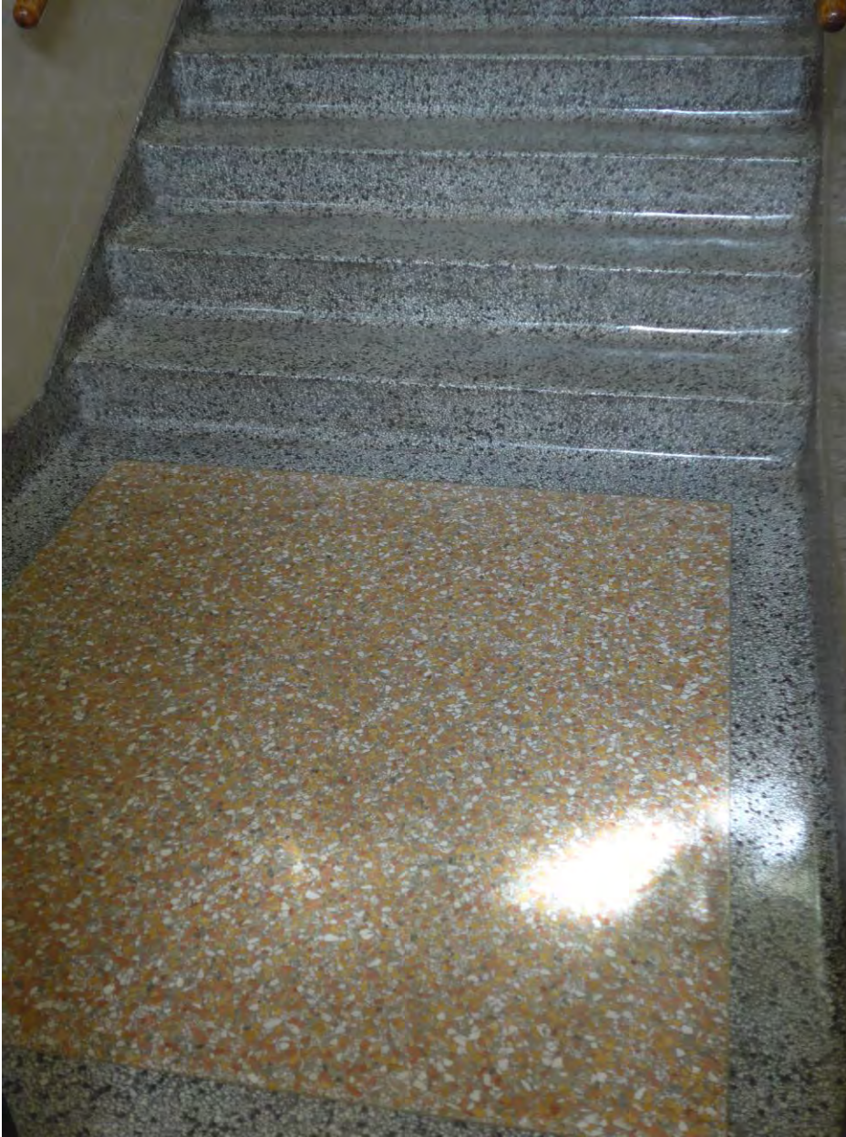
Interior detail view of terrazzo flooring, first floor stair hall 22 of 22
