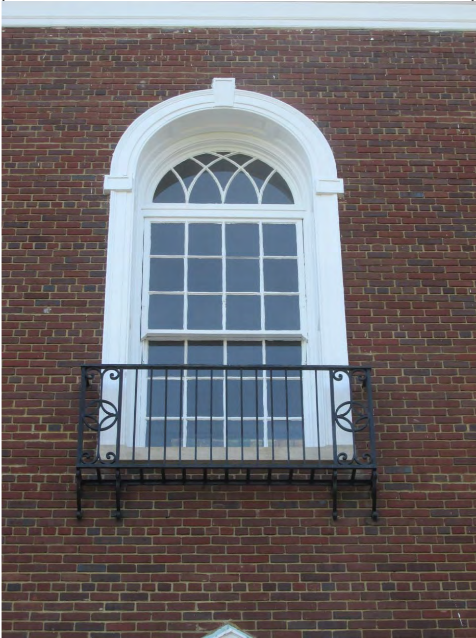
Detail of Palladian window at rear of building showing wrought iron railing that incorporates the Chinese coin motif
