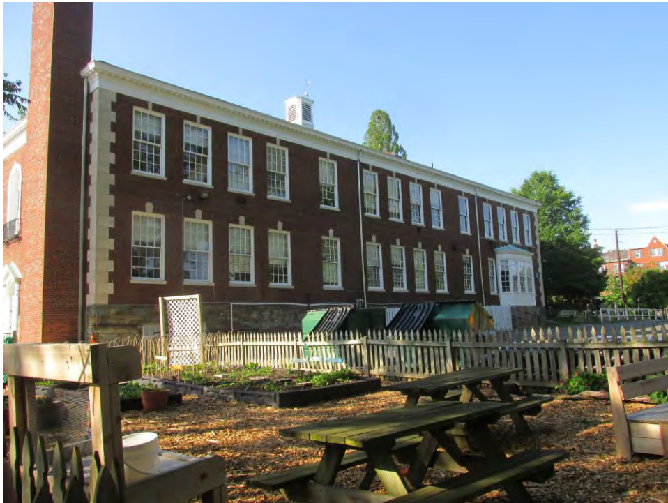
General view looking north from Hardy Recreation Center 4/22
