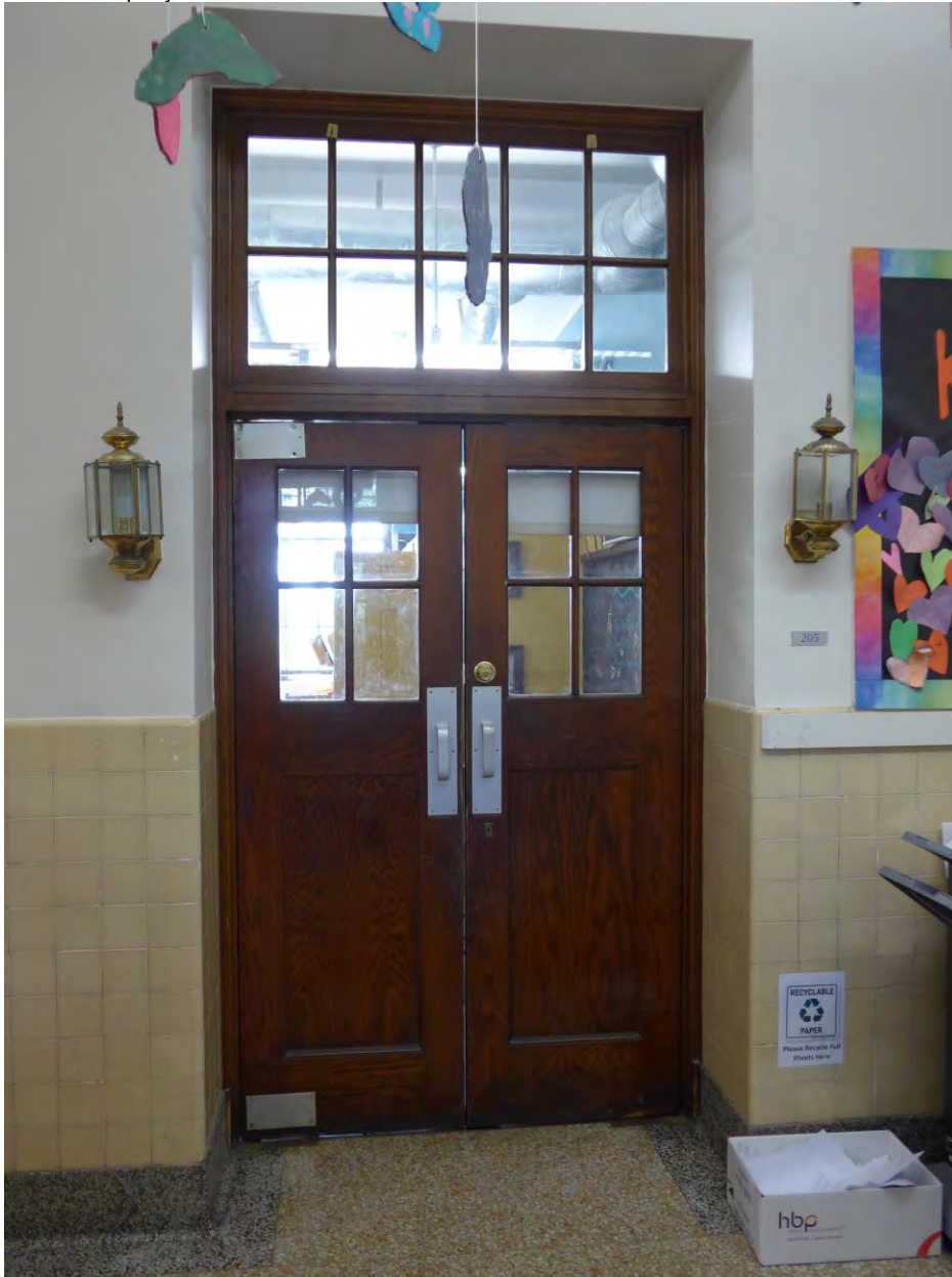
Interior view to classroom door in second floor corridor 19 of 22
