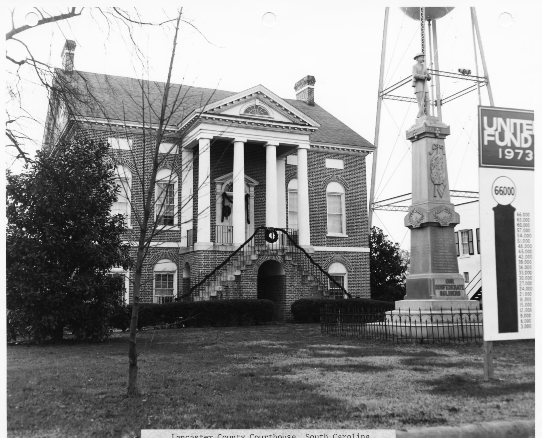
Lancaster County Courthouse, South Carolina
