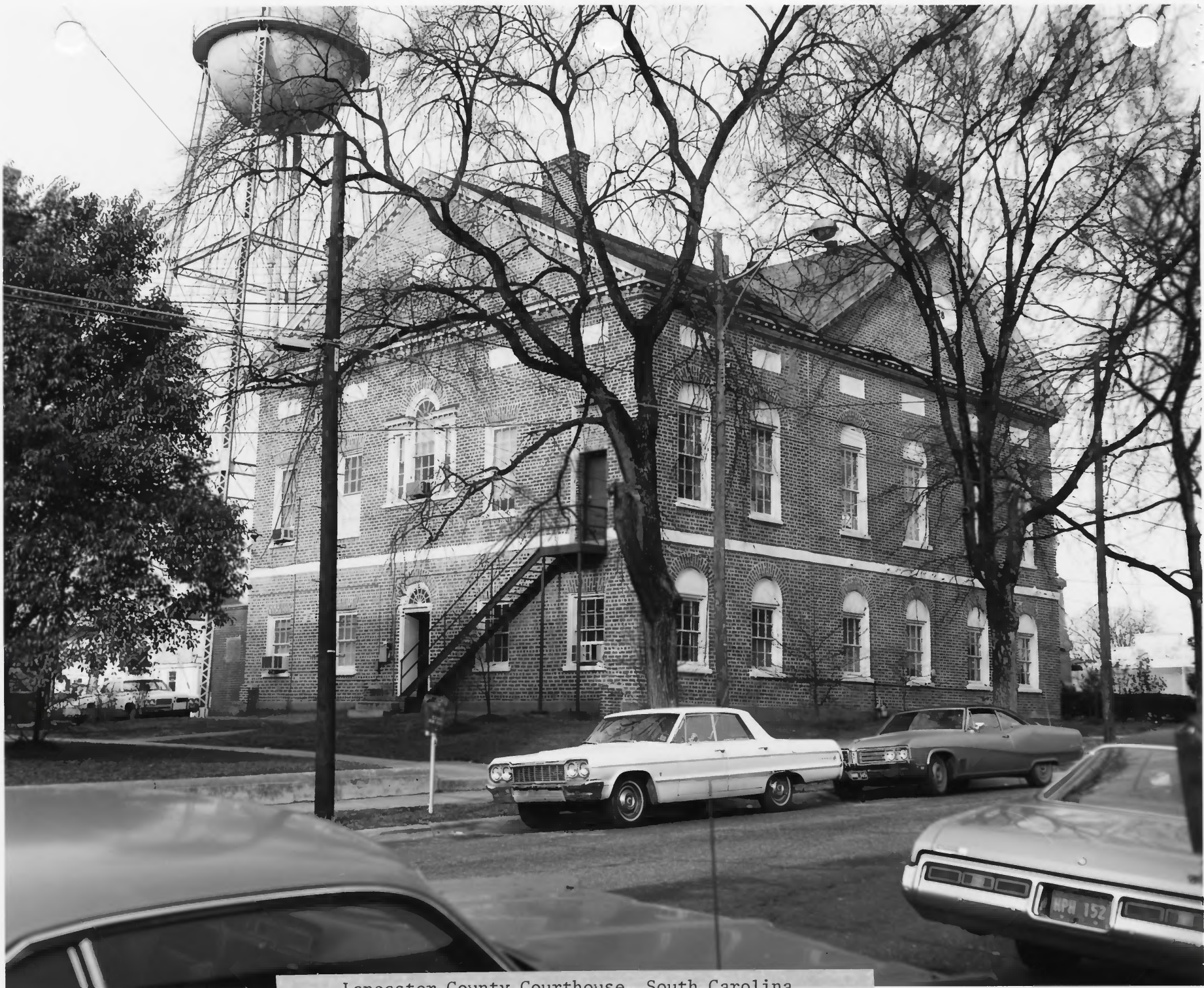
Lancaster County Courthouse, South Carolina
