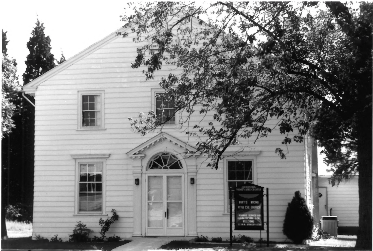
front facade (North) 034/011
