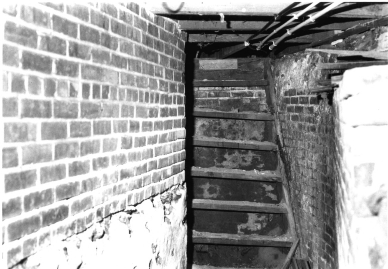
old stairwell (now closed off) 034/011 14 of 14
