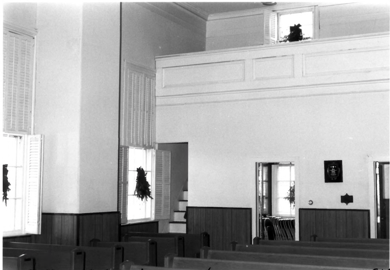
North west interior 034/011
