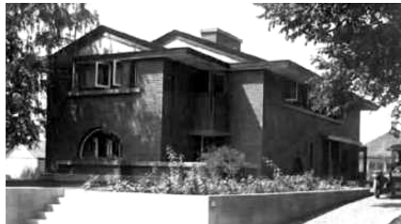
Image O Dr. Clarke House (built 1915-1916), Fairfield, IA. Extant. 500 S. Main St. NR Listed 02/08/80.
