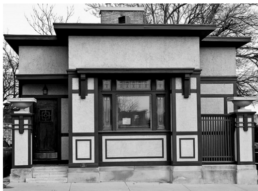
Image P Ernest M. Wood Studio (built 1912), Quincy, IL. Extant. 126 N. 8 th St. NR Listed 08/12/82.
