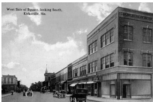
Image T The Odd Fellows Building (built 1913), is in the foreground on the far right. Kirksville, MO. (Pickler Memorial Library). Razed.
