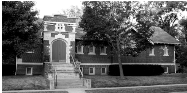
Image N Trinity Episcopal Church (built 1917), Kirksville, MO. Extant. 124 N. Mulanix St. NR Listed 01/02/08.
