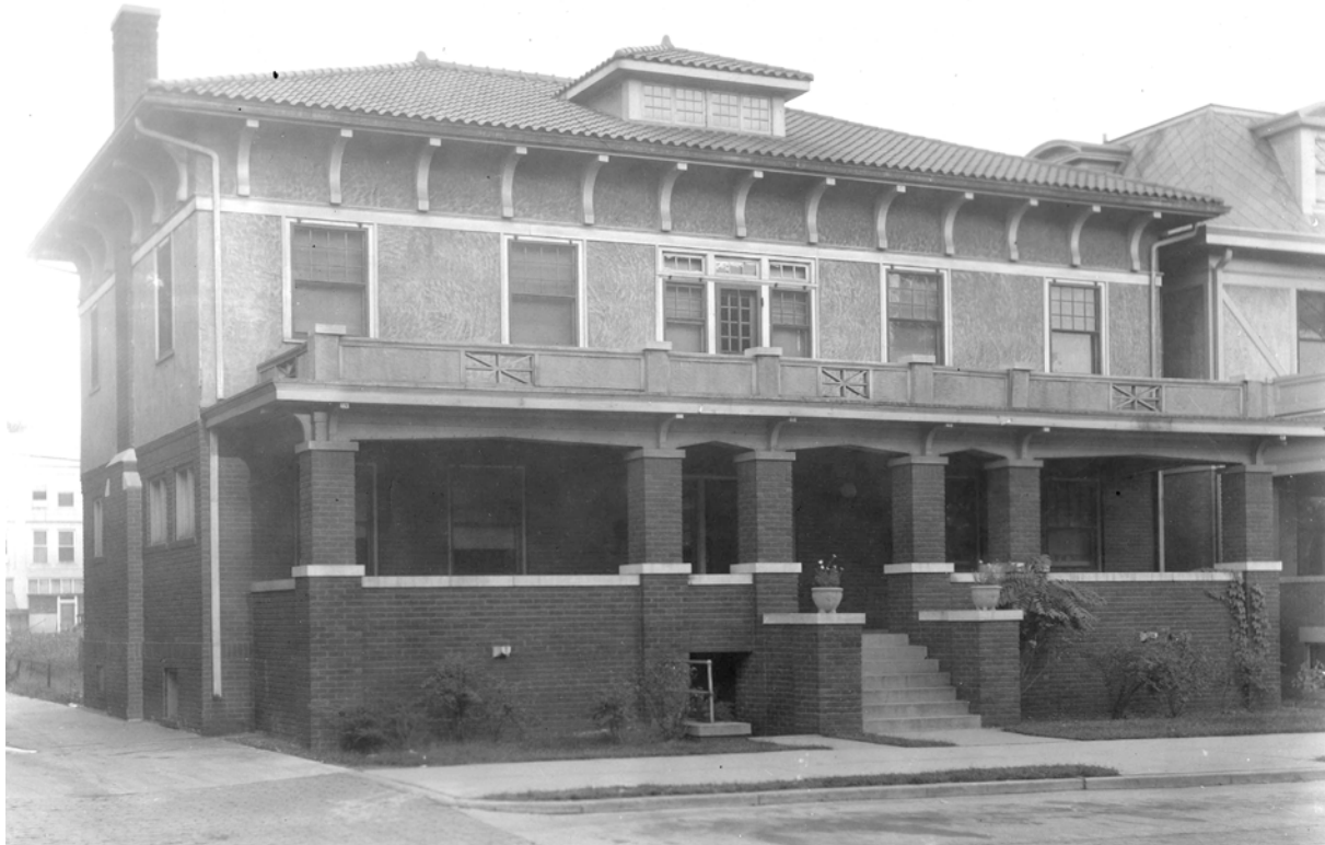
Image F Sojourners Club, West Façade, c. 1928. Note the original configuration of the veranda and second story terrace (closed balustrade) as well as the contrasting paint on the second story stucco and wood. (Truman State University).
