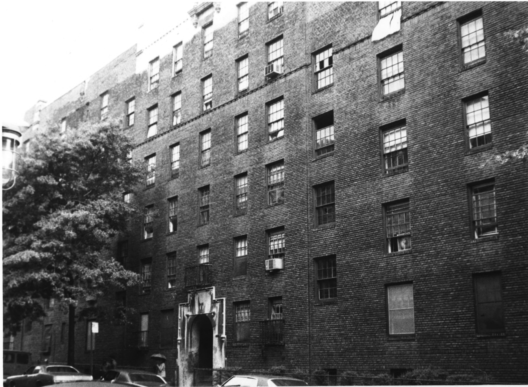
Matthew Henson Residence (Dunbar Apartments), 246 W. 150th Street, New York, New York Photo by ABC for NPS, 1974
