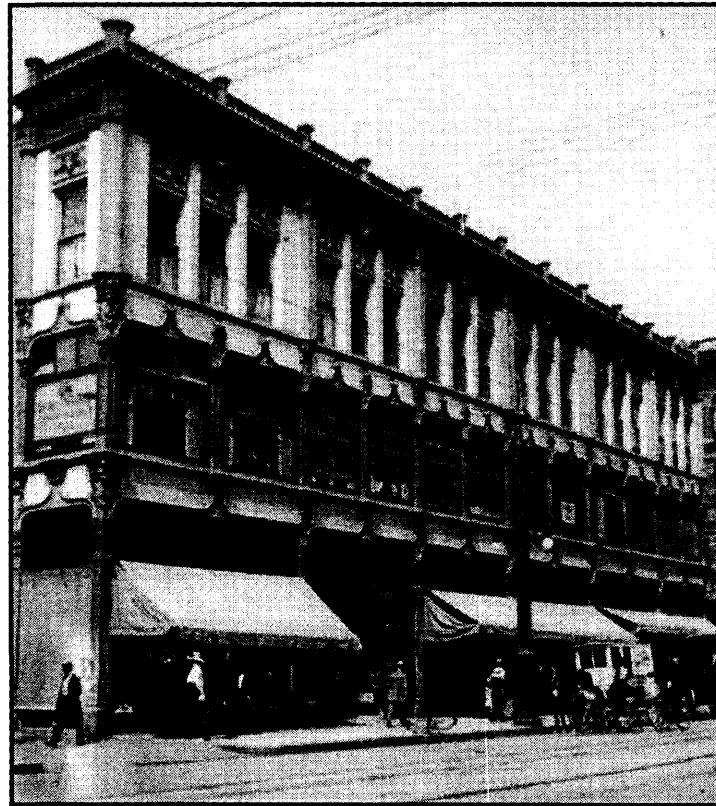
Figure 2. The 16 th Street side of the McClintock Building is shown here in about 1913. SOURCE: Denver Public Library, Western History and Genealogy Department, photographic collection, image X-18751.
