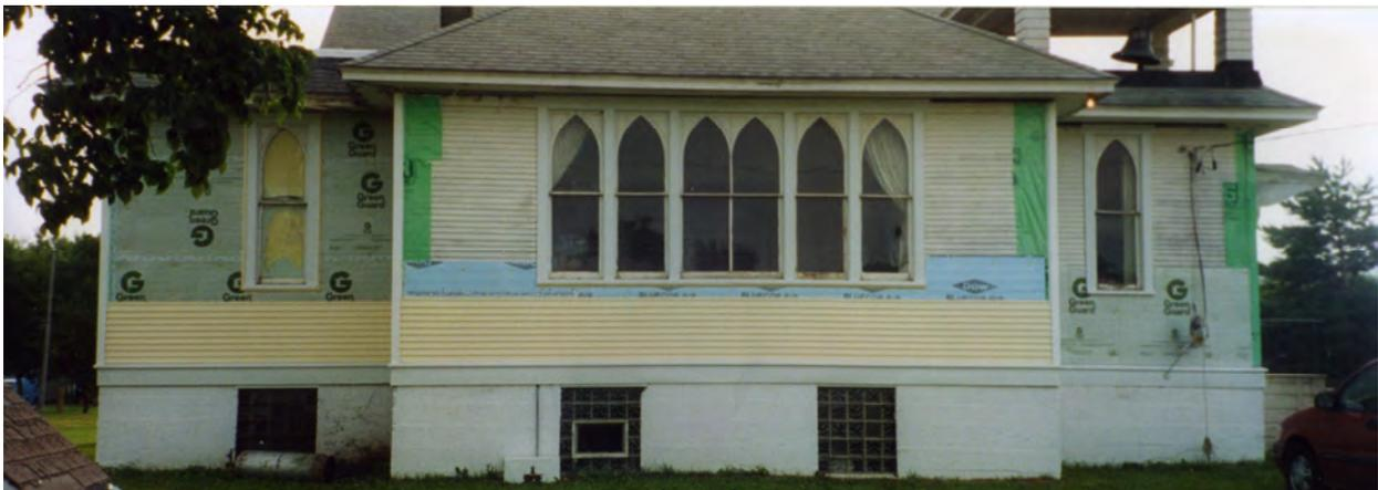
Figure #10 – Work on the siding and roof in 2002, showing both the old wood siding and new vinyl siding. Property of the Littleton and Chatham Historical Society.
