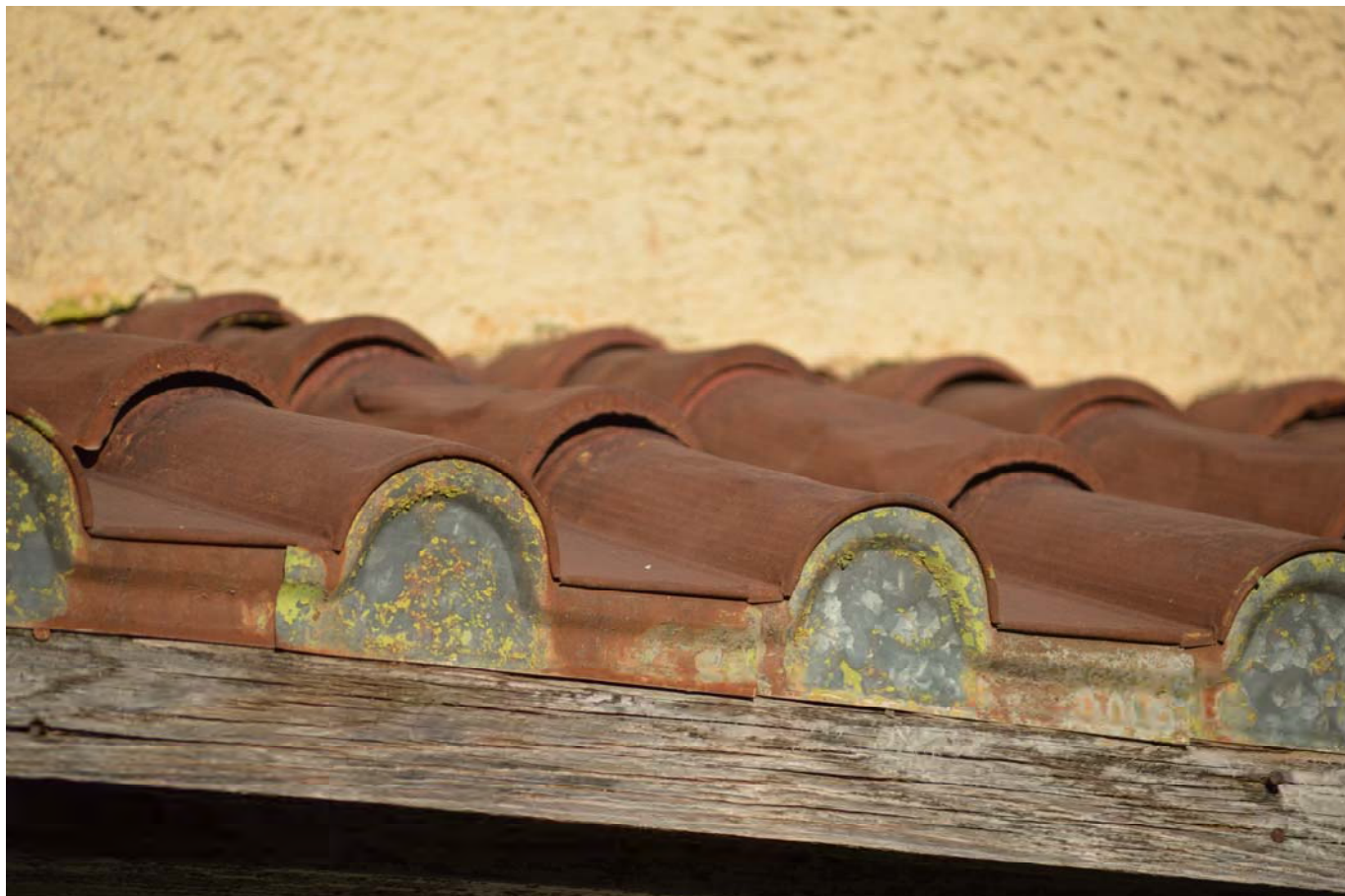
Photo 11 Metal roof cover detail
