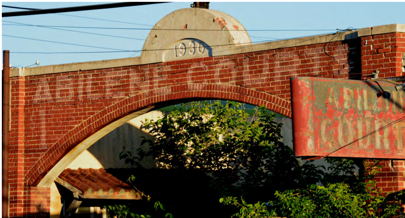
Photo 2 Archway over drive, camera facing southeast
