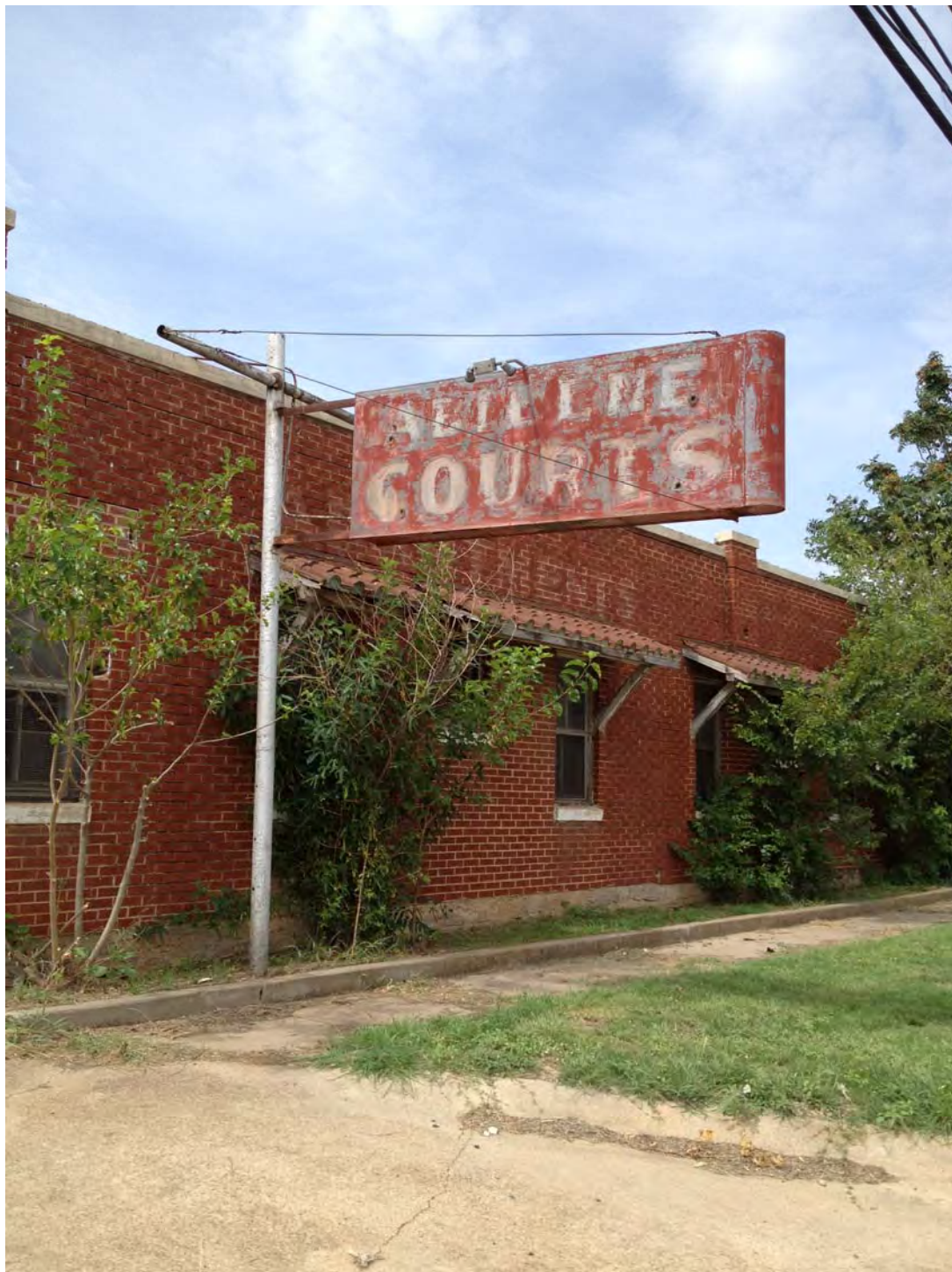
Photo 3: Neon sign and painted signage on south elevation. Camera facing southwest. Photographed by Gregory Smith, July 2013
