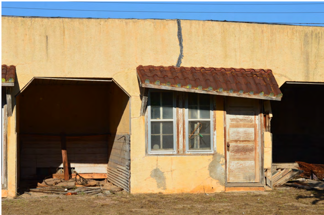
Photo 9 Open car bays, camera facing north
