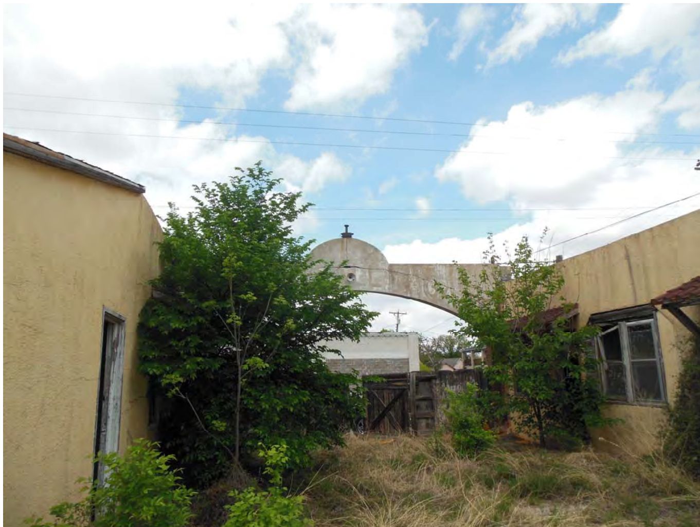
Photo 7 Entrance gate from courtyard, camera facing north Photographed by Stephanie Goodman
