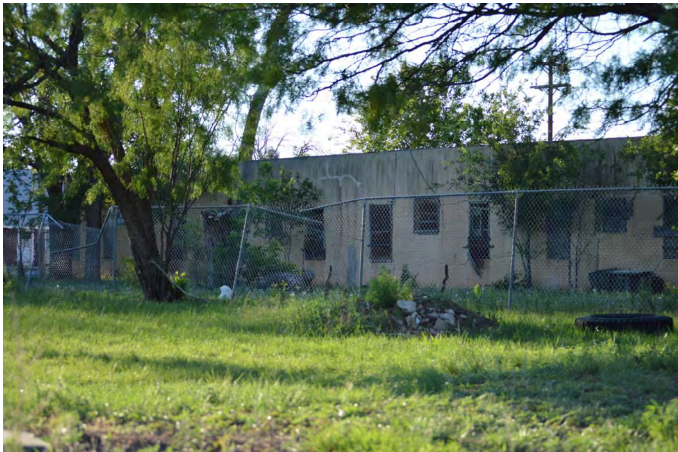
Photo 13 Southern façade, camera facing northwest
