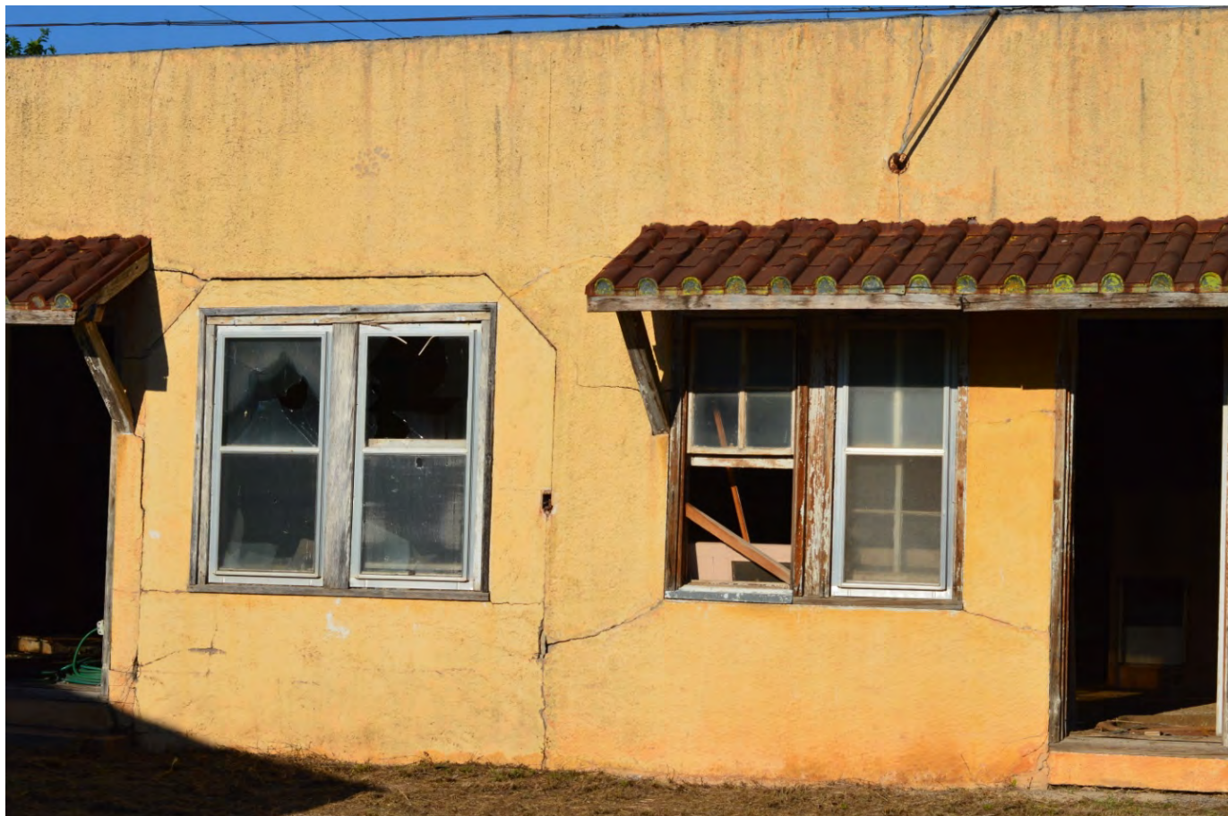
Photo 10 Open car bays, camera facing north
