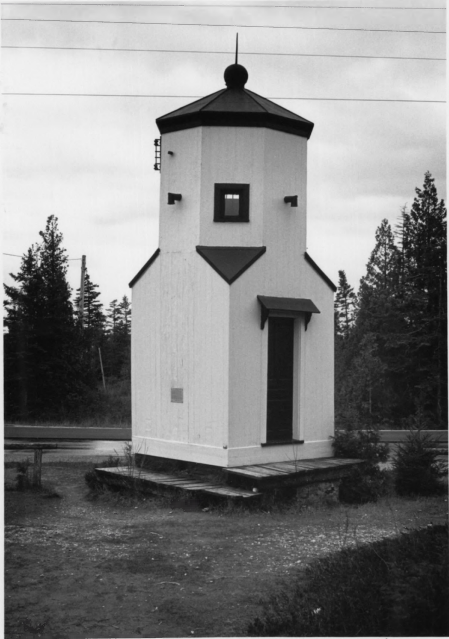
Baileys Harbor Range Lights, Door County, WI #4 of 5
