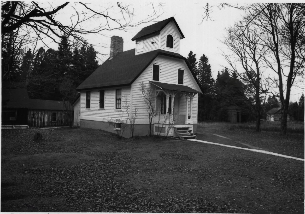
Baileys Harbor Range Lights, Door County, WI # 3 of 5
