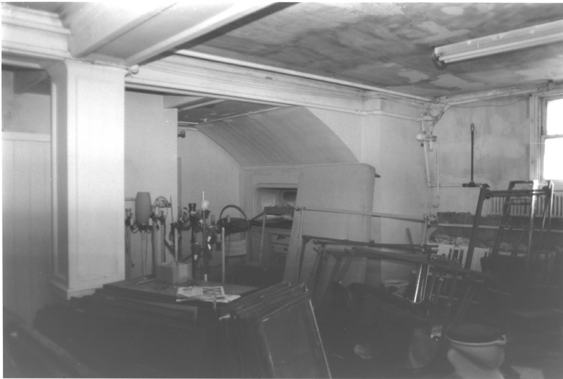
Ogden Apartment Hotel Minneapolis, Hennepin County, MN 010893 - 24A
