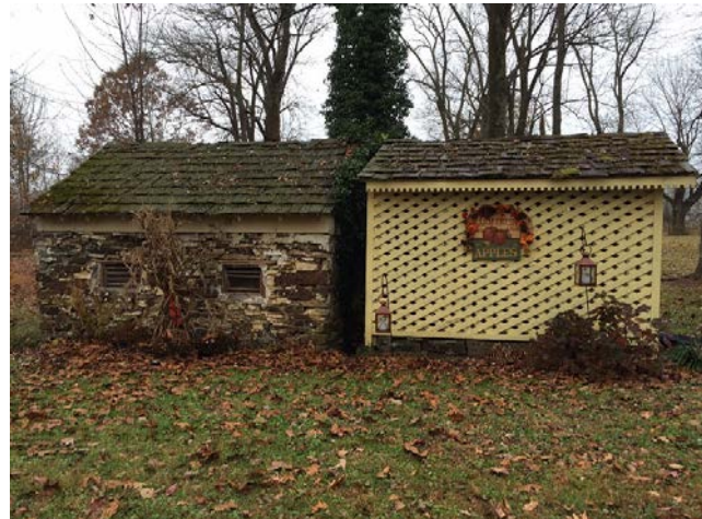
East side of Historic Springhouse and Frame Springhouse
