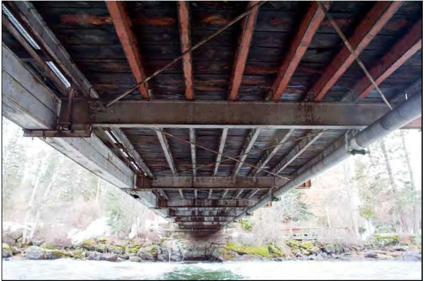
Photo 0007. Detail of underside of the bridge. View to the southwest.
