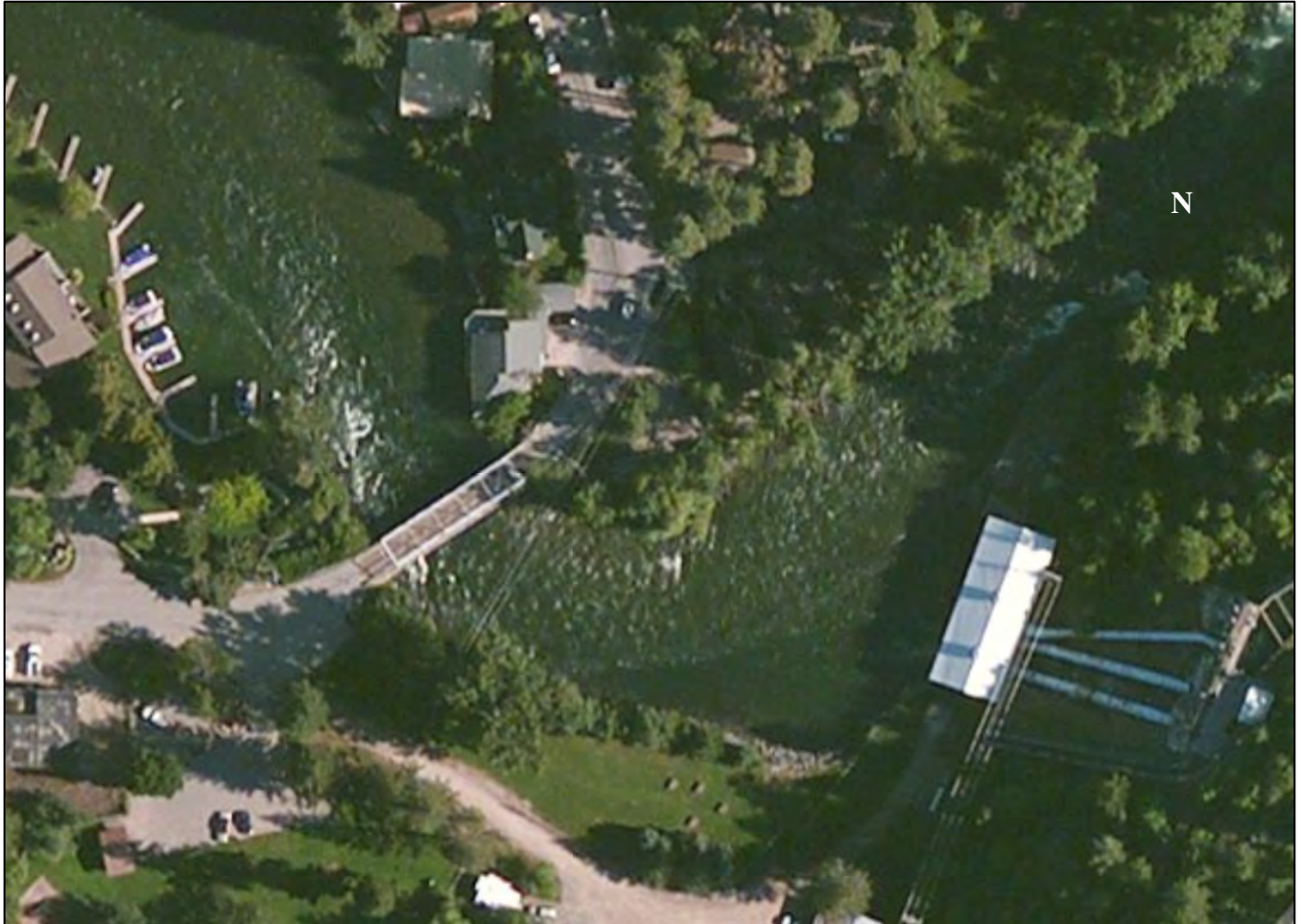
Aerial View of the Swan River Bridge.
