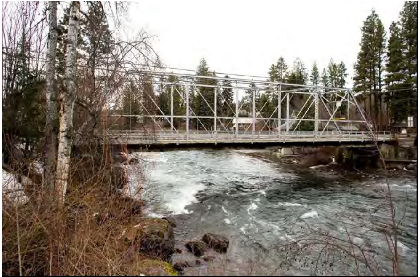
Photo 0002. Southeast side of the bridge. View to the northwest.
