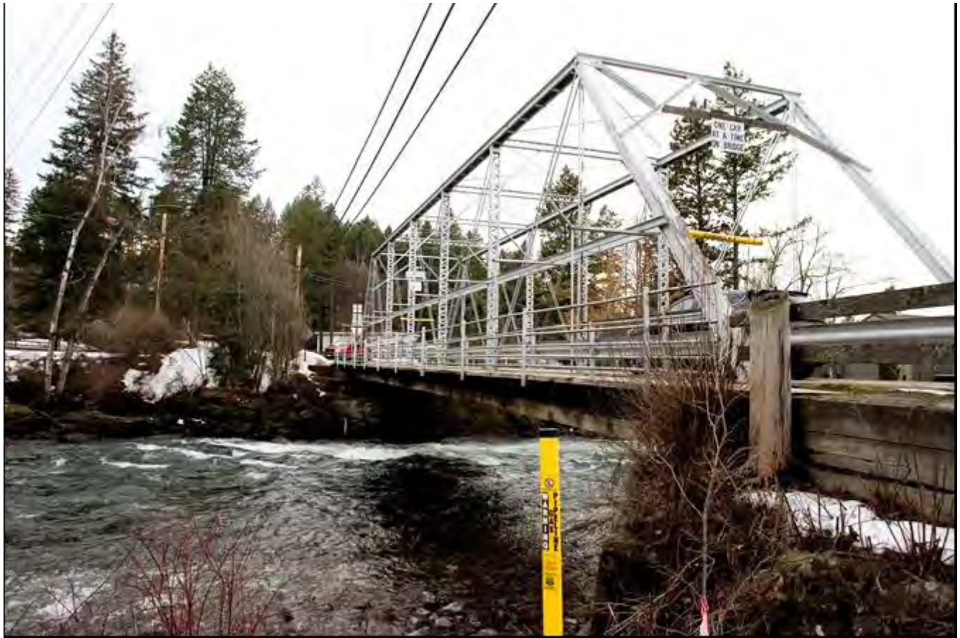
Photo 0004. Southeast side of the bridge. View to the northeast.
