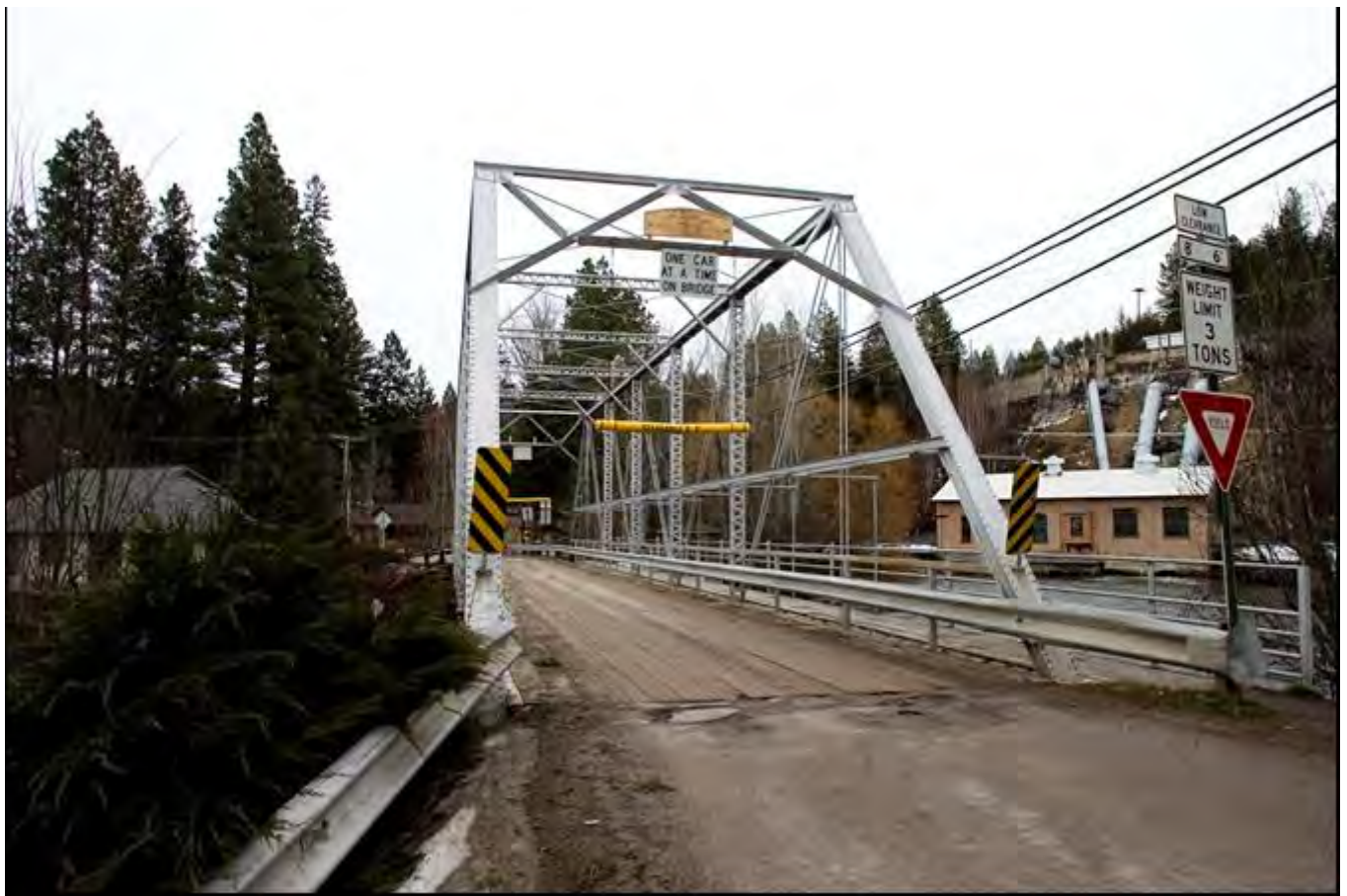
Photo 0005. Southwest portal of the bridge. View to the northeast.
