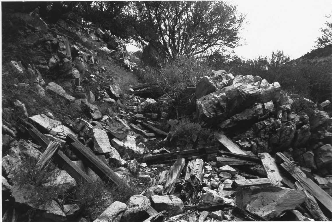
OSCEOLA (EAST) DITCH, WHITE PINE, NEVADA (PHOTO #1)
