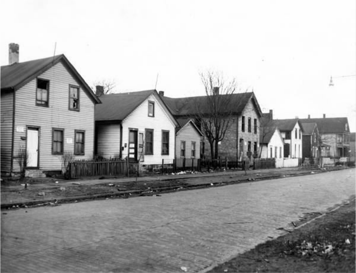
Figure 7: Cedar-Central Neighborhood, 1953; These houses were demolished as part of slum clearance for the construction of the Cedar-Central Apartments Extension. Michael Schwartz Library, Cleveland State University.
