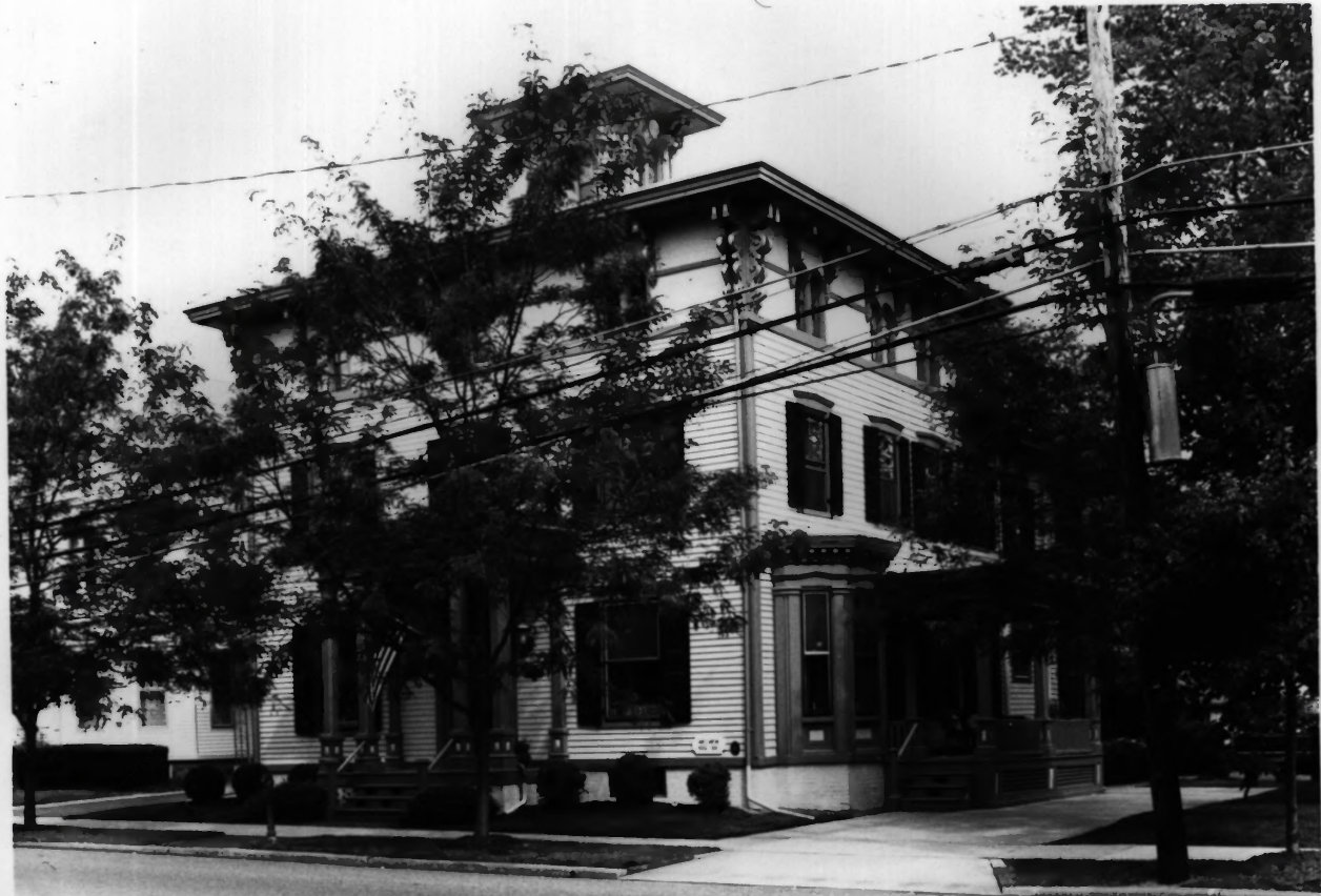
James + Mary Lawson House, Salem County, New Jersey Photo # 2
