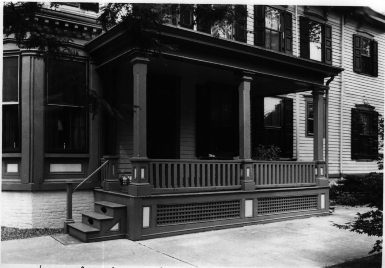
James + Mary Lawson House, Salem County, New Jersey Photo #9
