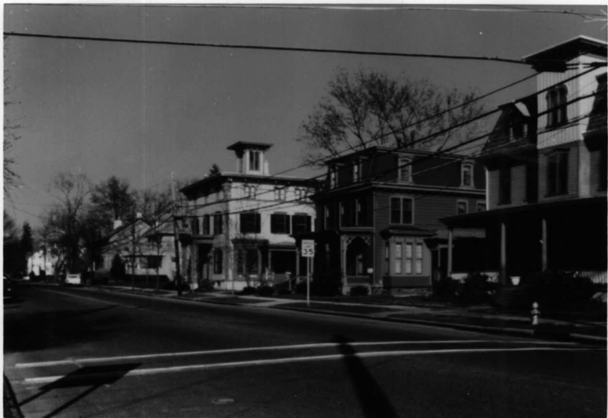
James + Mary Lawson House, Salem County, New Jersey Photo #5
