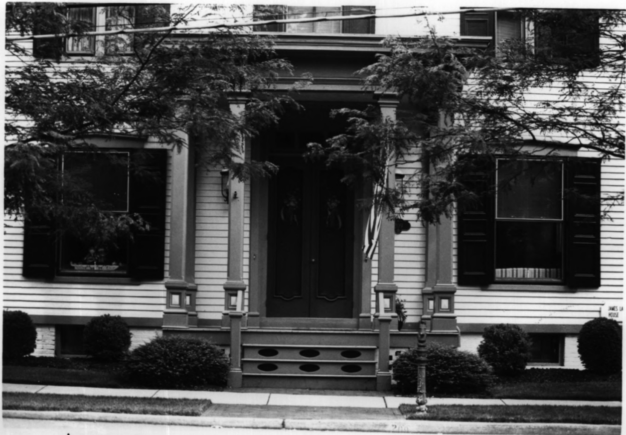
James + Mary Lawson House, Salem County, New Jersey Photo # 7
