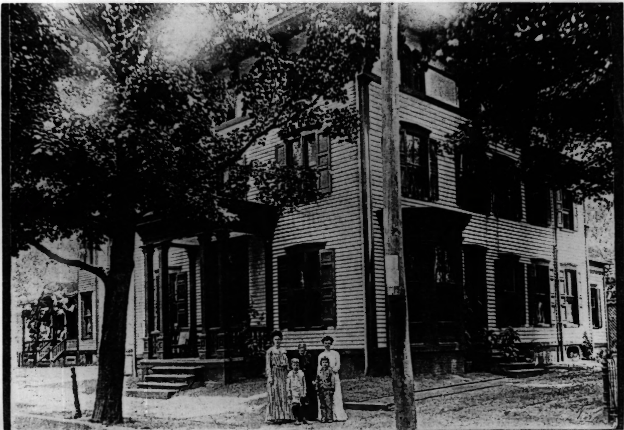
James & Mary Lawson House, Salem County, New Jersey Photo #17
