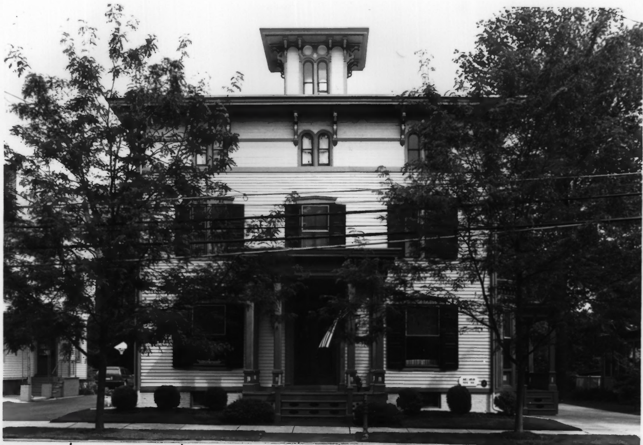
James & Mary Lawson House, Salem County, New Jersey Photo #1
