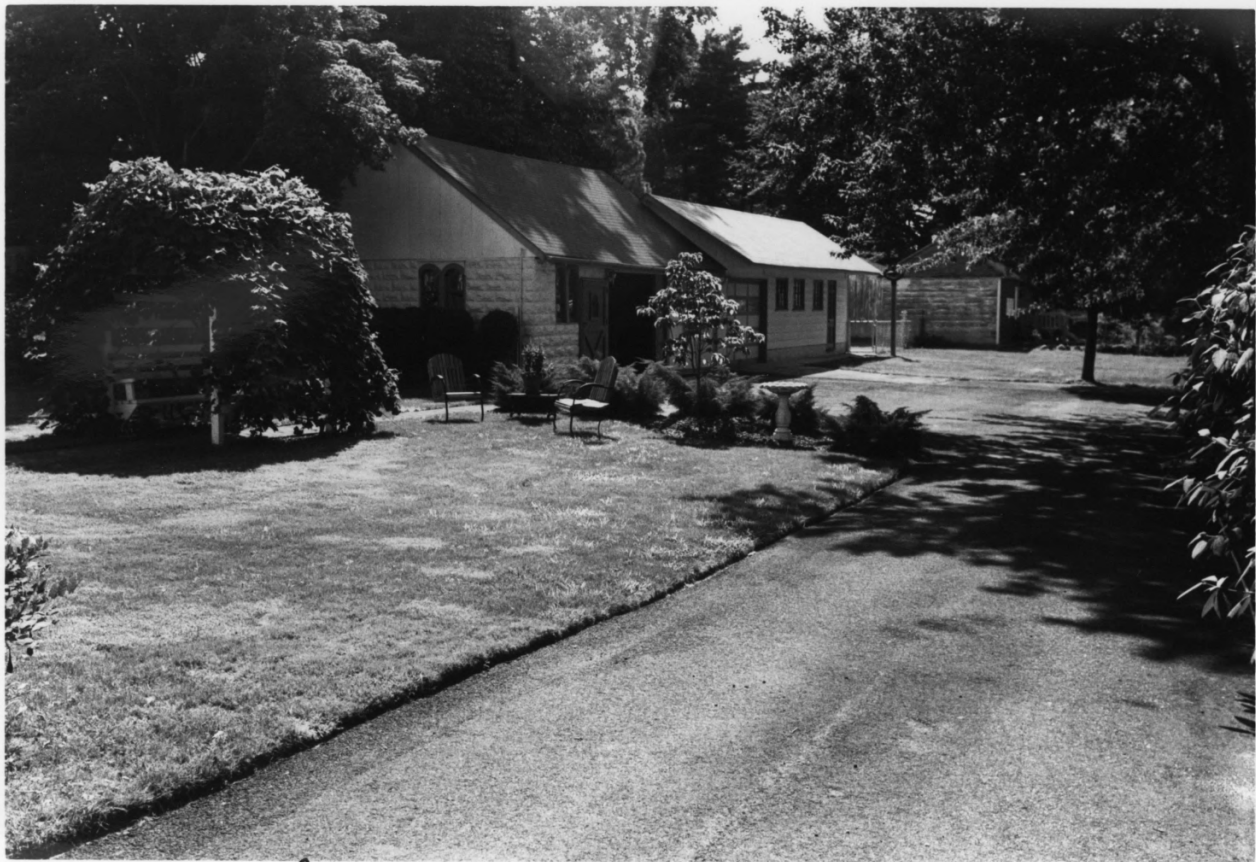
James + Mary Lawson House, Salem County, New Jersey Photo #12
