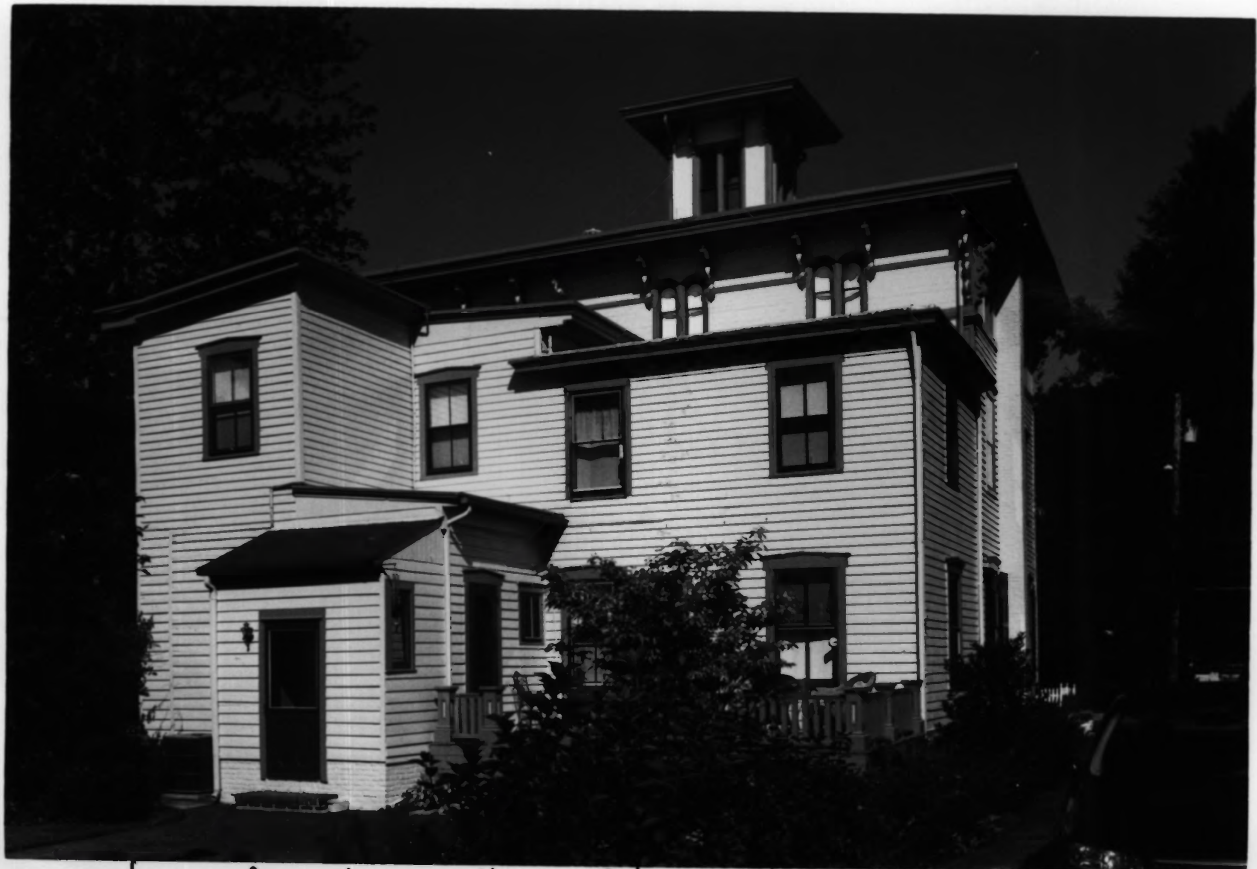
James + Mary Lawson House, Salem County, New Jersey Photo # 4
