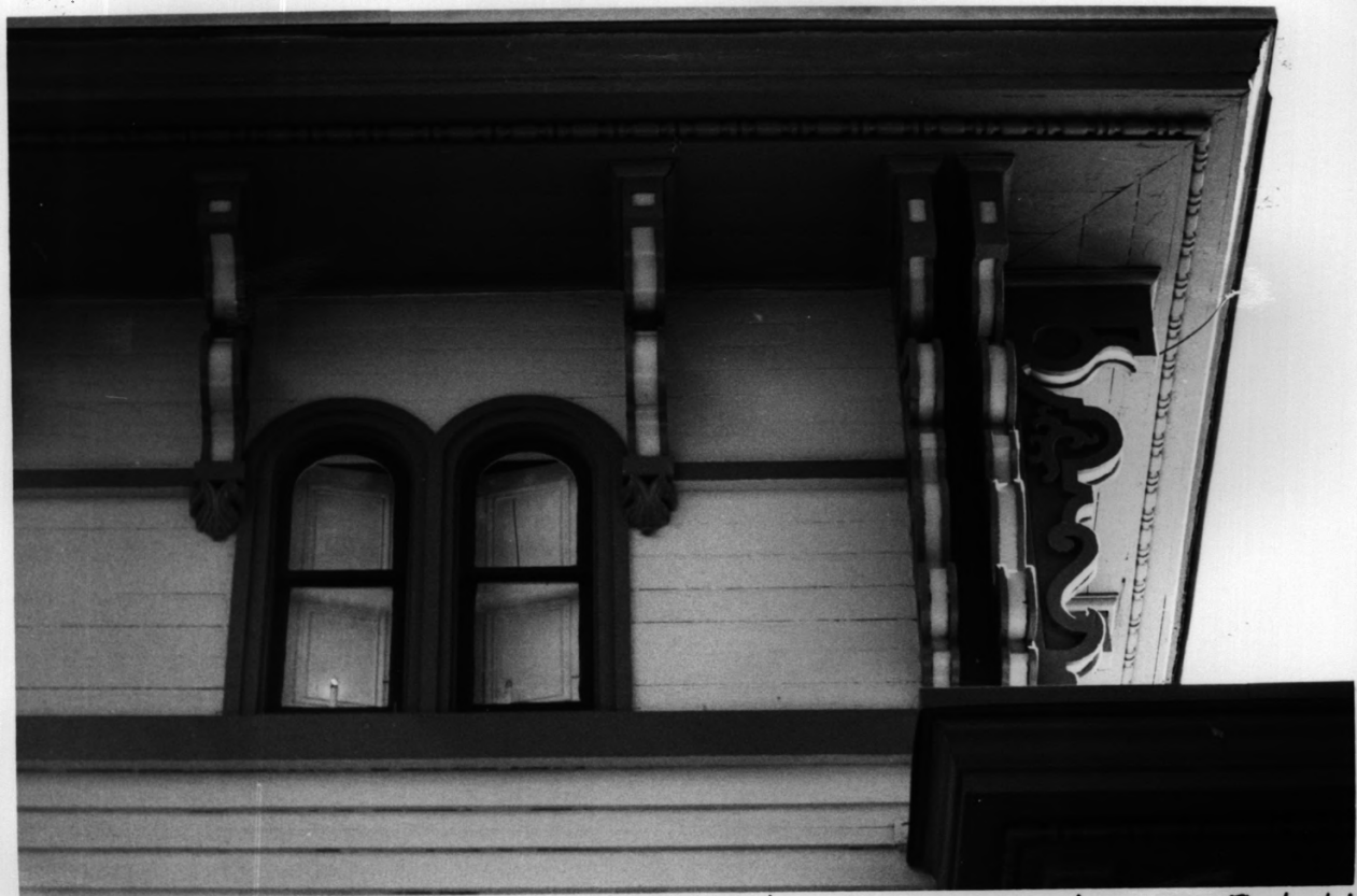
James + Mary Lawson House, Salem County, New Jersey Photo # 11
